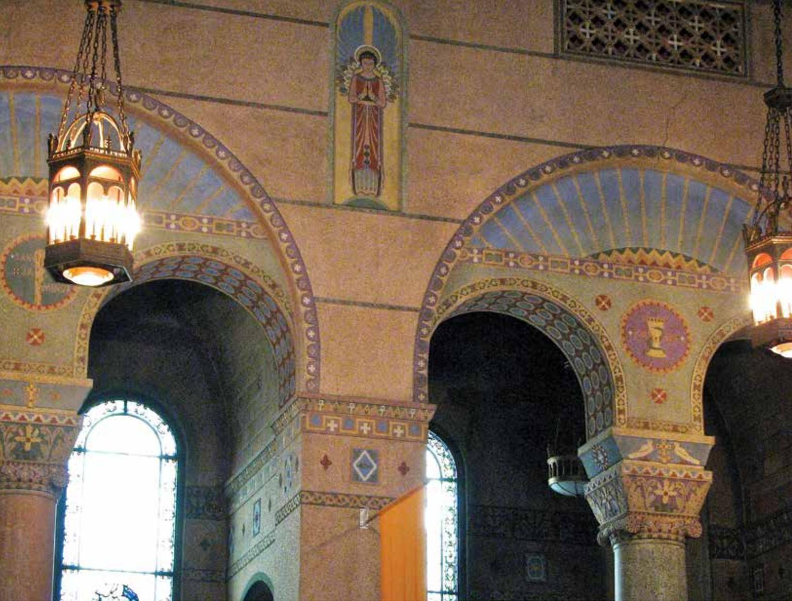
**Fig. 1: John Earley stunned the industry in 1921 by creating breathtaking colors, forms, and textures with exposed aggregate polychrome mosaic concrete for the interior of the Shrine of the Sacred Heart, Washington, DC. For architectural decoration and moldings, Earley Studio installed polychrome mosaic concrete as thin, precast slabs and applied stucco with great precision. About 200 colors of aggregate were crushed and sieved into pebbles and sand before combining them in concrete mixtures**
