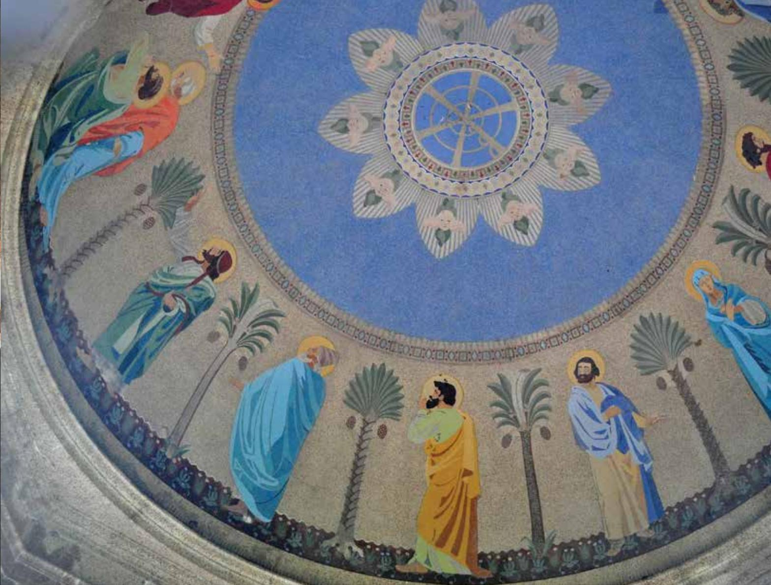
**Fig. 2: The dome of the open-air Chapel of the Ascension at the Franciscan Monastery, Washington, DC. Thin, precast slabs were prepared on curved molds in the studio for the figures, trees, and decoration. The thin, precast slabs were installed on the dome with a brown coat before mosaic stucco was applied by trowel onto the tan and blue background areas**
