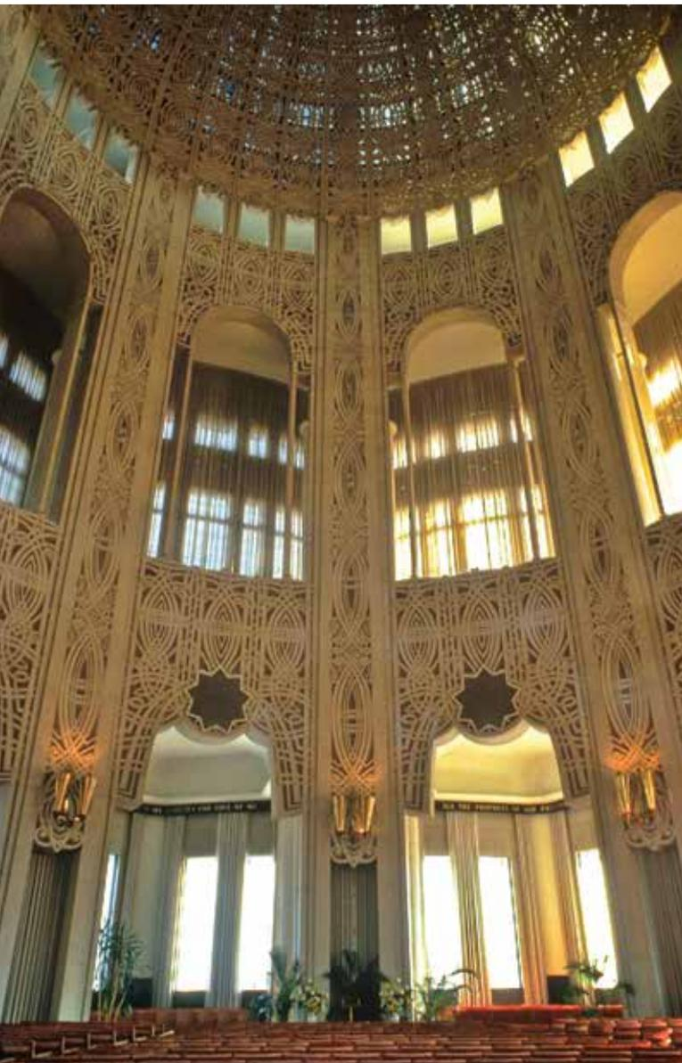
Fig. 3: The Bahá'í Temple interior displays 2457 panels of polychrome precast mosaic concrete with ornamentation sculpted in 2 in. (50 mm) deep relief
