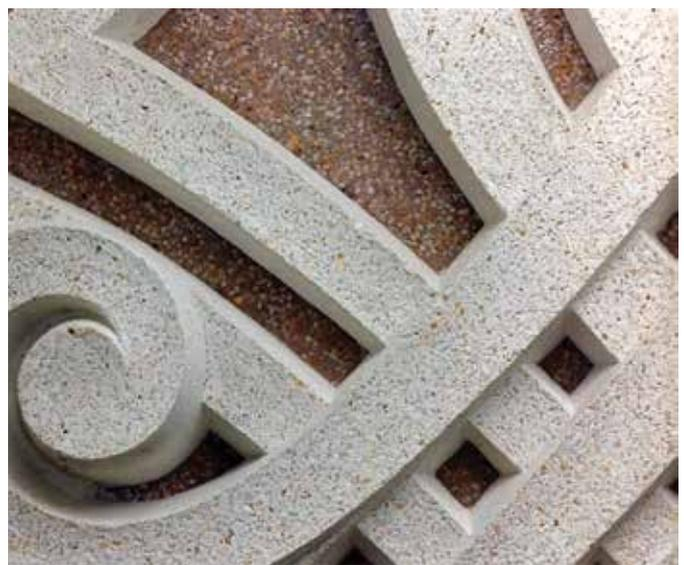
Fig. 4: Closeup of concrete panels for the Bahá'í Temple. Panels display remarkable precision in delineation of the color, sharp arrises, uniform exposure of the aggregate, and a third chroma effect by not exposing the sides
