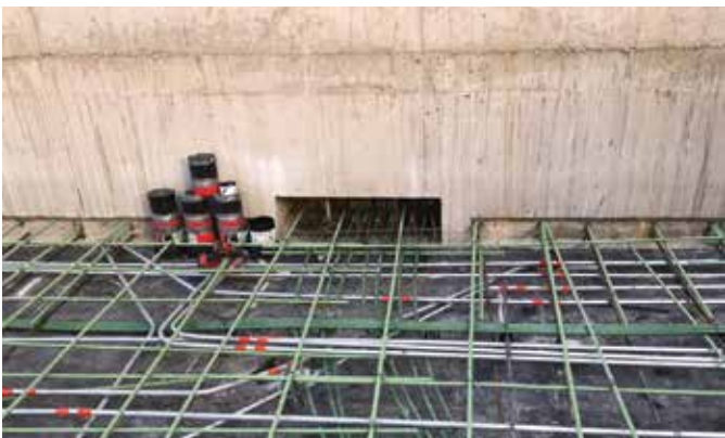
Fig. 5: Blockout in structural wall for stressing-end anchors. Backup bars are not shown (photo courtesy of James McHugh Construction Co.)
