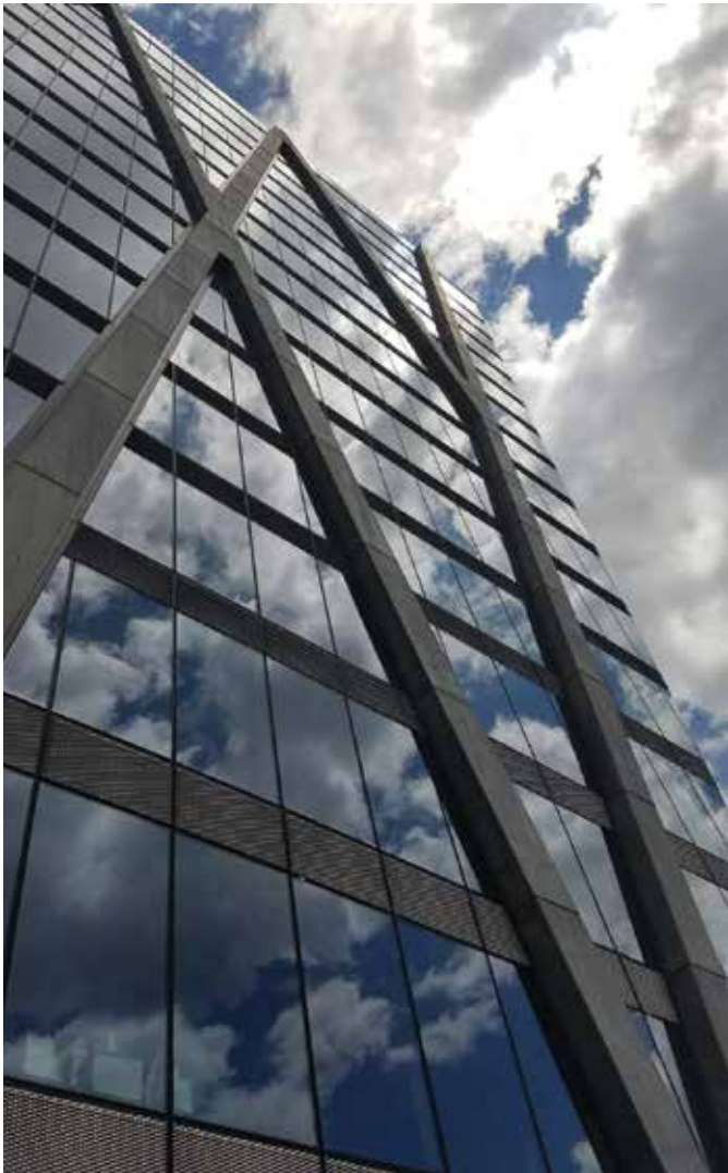
Fig. 5: The exposed concrete exoskeleton columns act as both braced frames and moment frames
