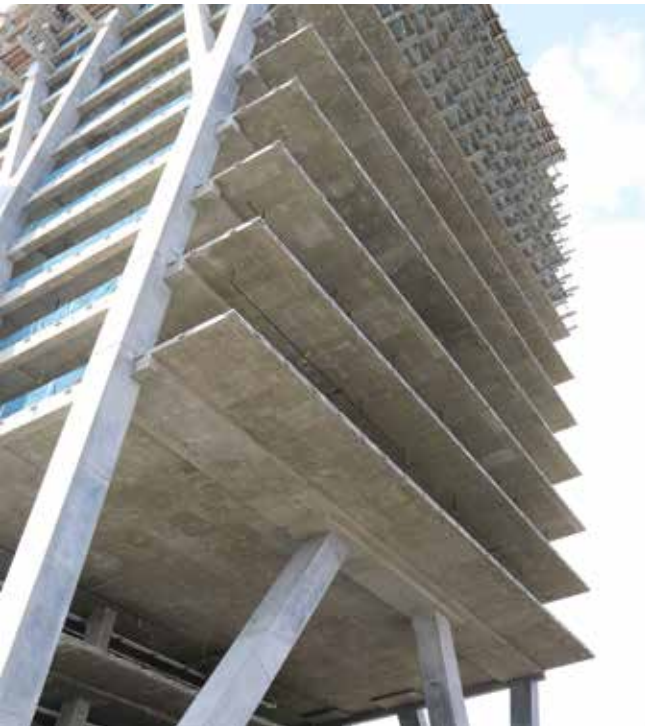
Fig. 3: Each floor slab has 15 ft (4.6 m) cantilevers in the north and south directions
