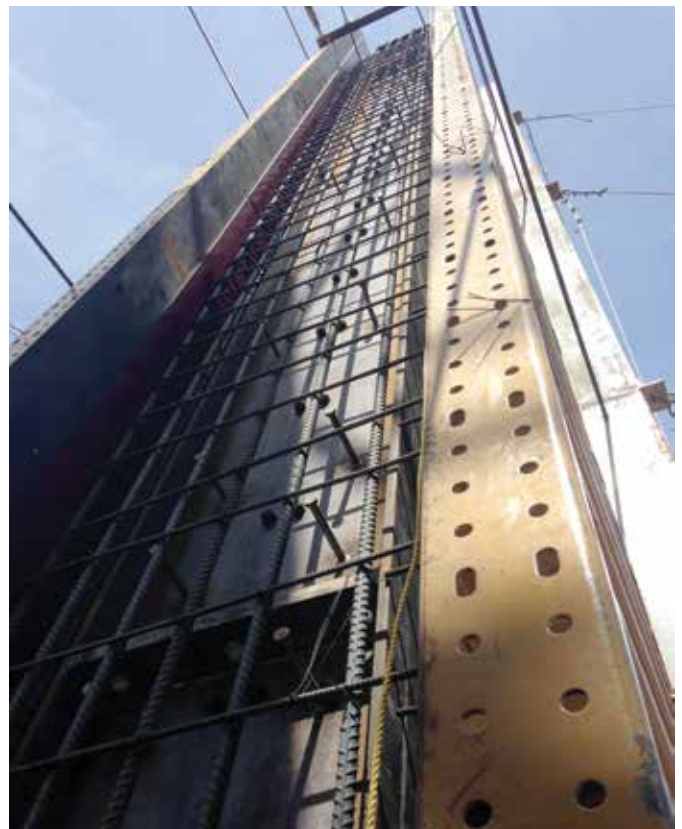
Fig. 7: Built-up structural steel core and deformed bars inside a tree column form (photo courtesy of DAVIS)
