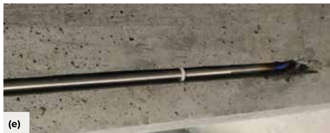
Fig. 4: Installation of titanium bars on the Mosier bridge: (a) grooves were cut using a diamond blade; (b) after holes were drilled and cut surfaces cleaned, epoxy was placed in the groove; (c) titanium “staples” were produced by bending hooks, shown here with a characteristic blue color where they had been heated for bending; (d) staples were inserted in the prepared grooves and holes; (e) close-up of the installation; and (f) after another layer of epoxy was applied to cover the staples, the girders were painted to complete the installation (photos courtesy of ODOT and Perryman Company)
