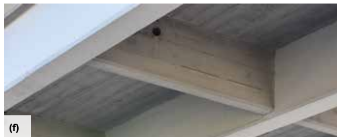
Fig. 4: Installation of titanium bars on the Mosier bridge: (a) grooves were cut using a diamond blade; (b) after holes were drilled and cut surfaces cleaned, epoxy was placed in the groove; (c) titanium “staples” were produced by bending hooks, shown here with a characteristic blue color where they had been heated for bending; (d) staples were inserted in the prepared grooves and holes; (e) close-up of the installation; and (f) after another layer of epoxy was applied to cover the staples, the girders were painted to complete the installation (photos courtesy of ODOT and Perryman Company)
