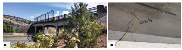
Fig. 2: The Mosier bridge is an overpass for a secondary road crossing I-84 in Oregon: (a) overall view of structure; and (b) cracks were observed near cutoff points for flexural reinforcement (photos courtesy of ODOT)
