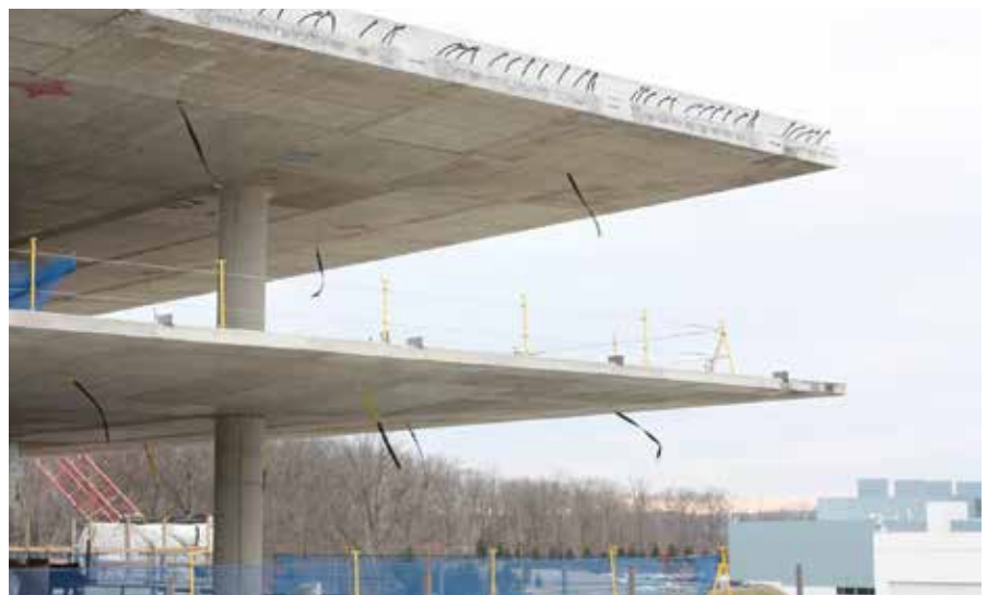
Fig. 5: View of 40 ft (12 m) cantilever at corners
