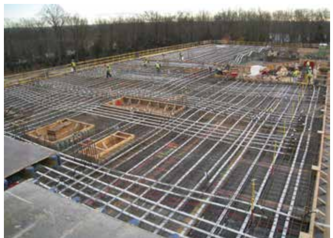
Fig. 2: Workers place PT tendons in a floor slab
