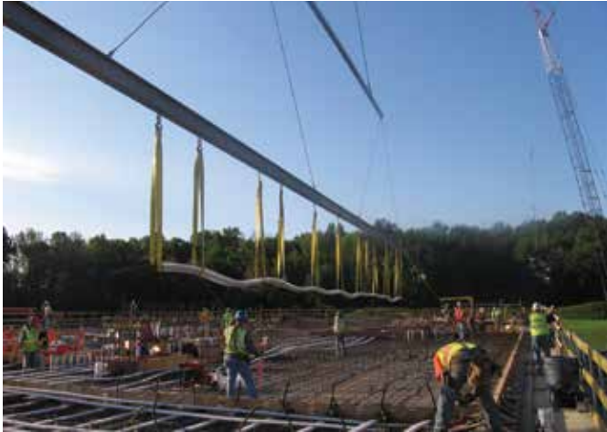
Fig. 10: Tendons were assembled and then lifted onto the slab formwork
