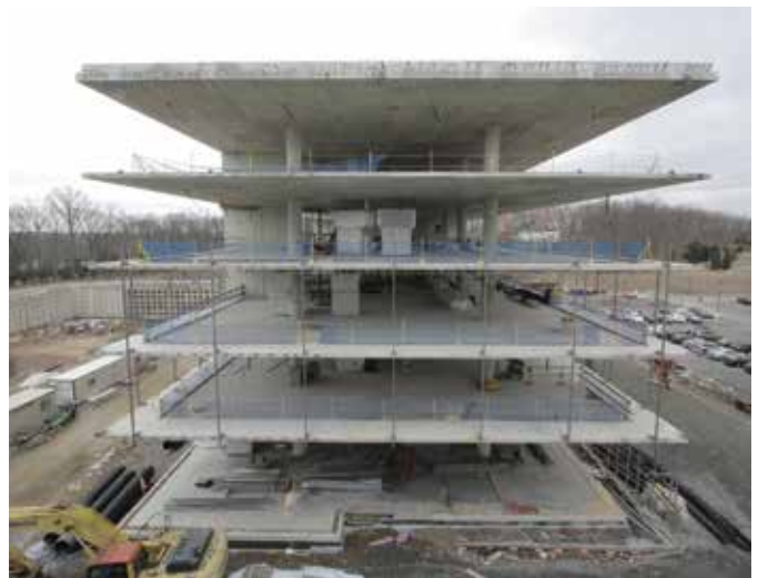
Fig. 1: View of the Novartis Oncology Research Building during construction
