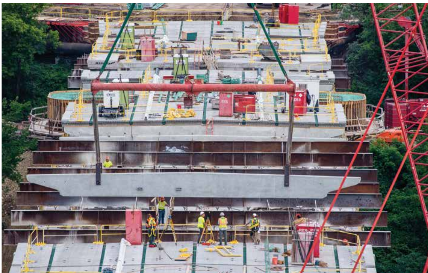
Fig. 8: An overview of the ABC process. In the foreground, a new cap beam is being placed. New deck panels are already in place in adjacent spans (photo courtesy of HNTB Corporation and Joe Szurszewski Photography LLC)
