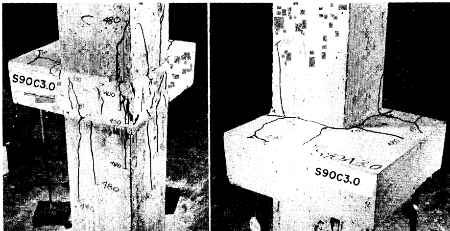
Fig. 10—Typical cracking for corner column specimens, Type C (slab series)
