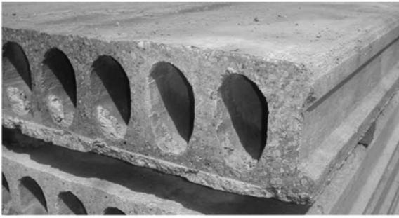
Fig. 1 The keyed edge profile of the hollow core units.
