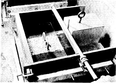
Fig. 2. - Forms Prepared for Slab Casting.
