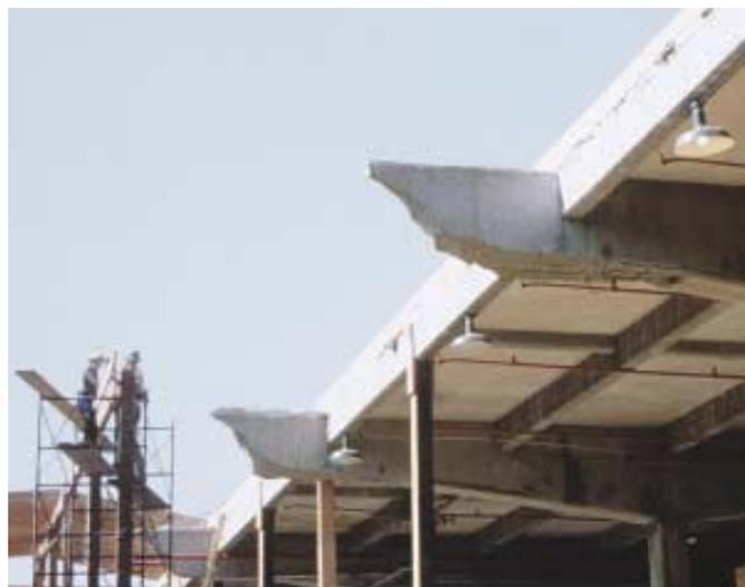
Fig. 2: Shear failure of 36-in.-deep (900 mm) beams in Air Force Warehouse, Shelby, OH (Photograph courtesy of Chester P. Siess)
