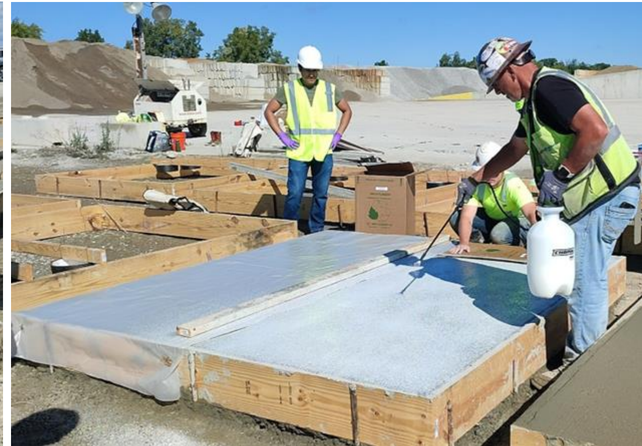
Application of curing compound
