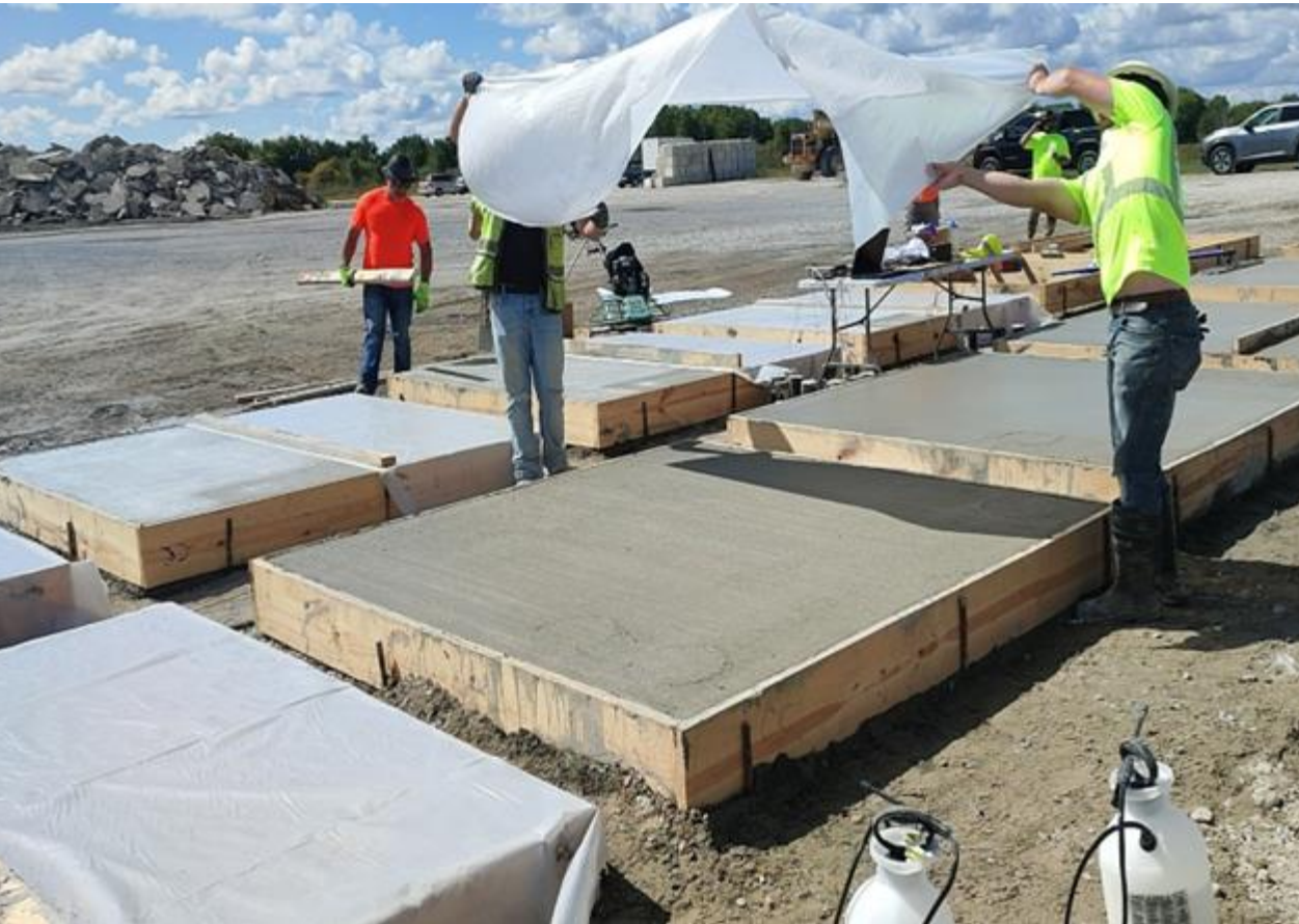
Placing plastic sheet over concrete
