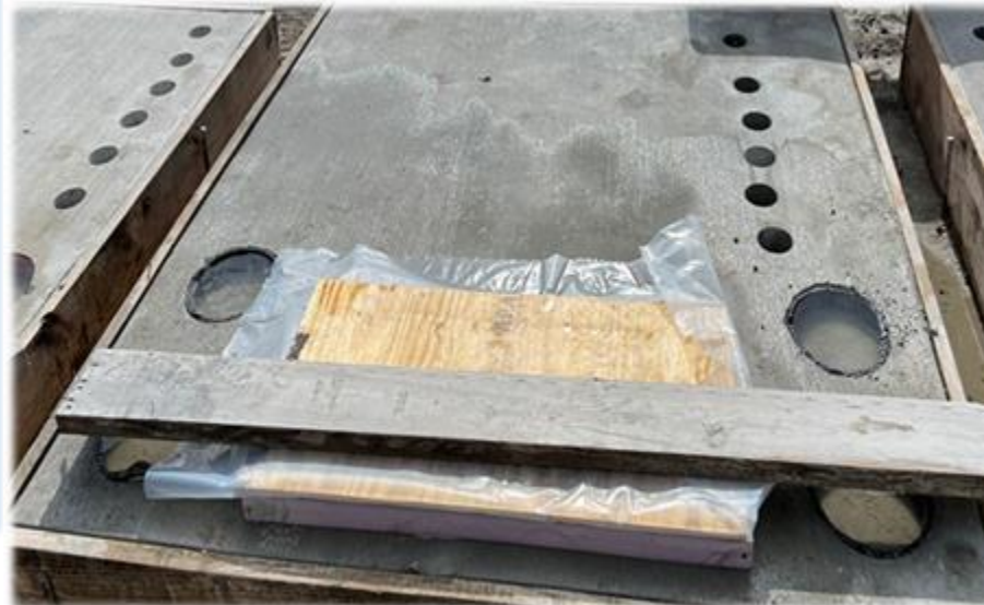
Covering dikes to avoid evaporation
