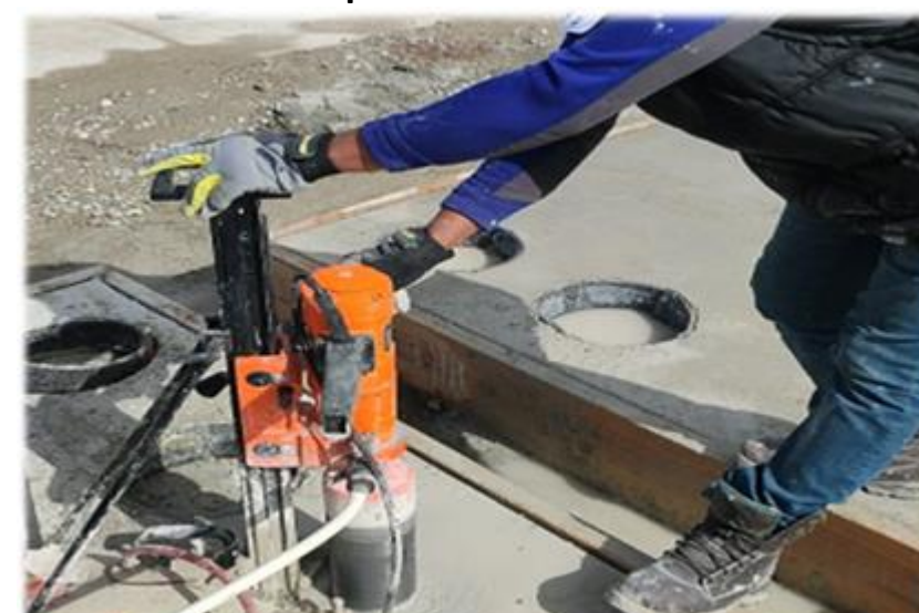
Extraction of concrete cores from the field
