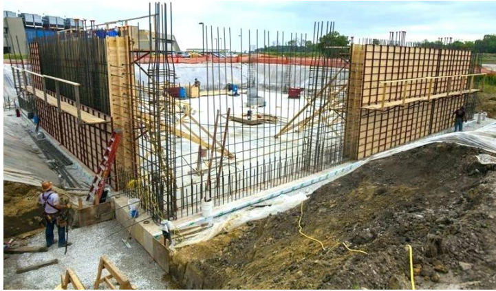
Conventional Construction (forming, reinforcement placement & casting)
