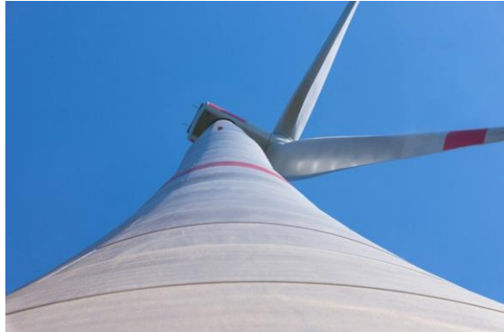
Onshore wind turbine concrete towers
