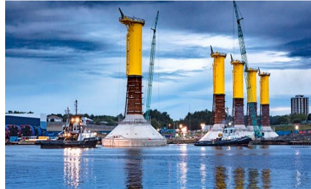
Offshore wind turbine concrete fixed base foundations
