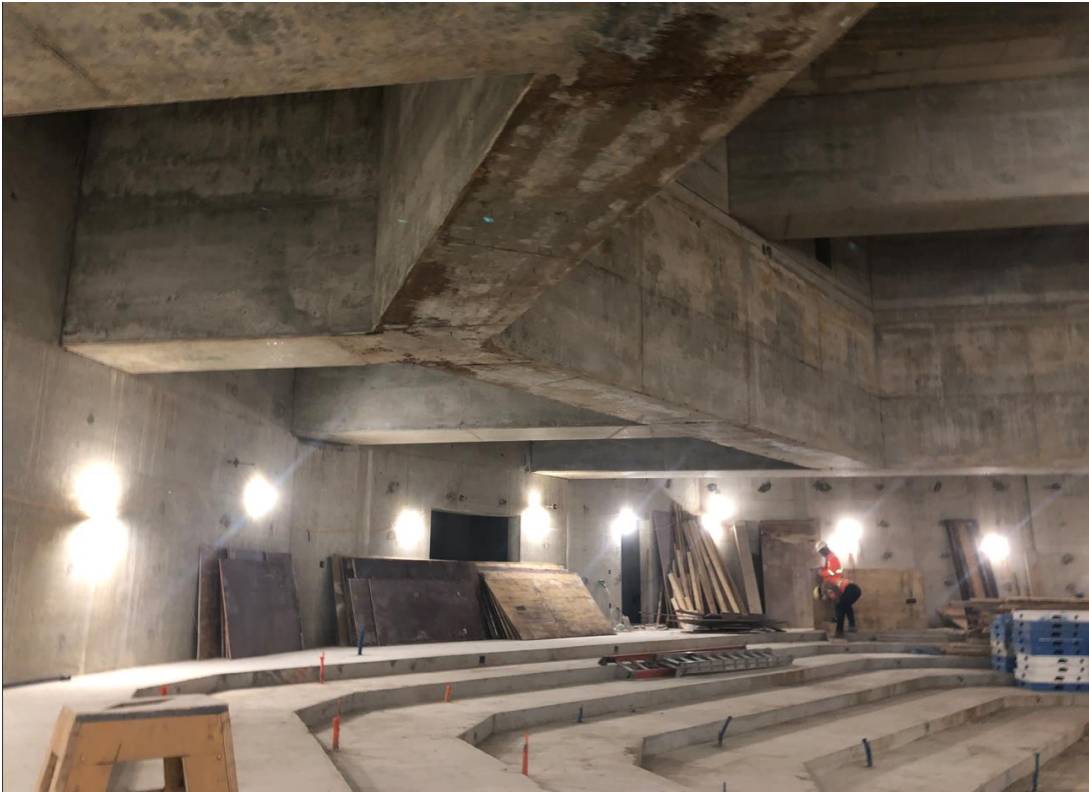
Supporting stage 1 beams framed to Ring Structure
