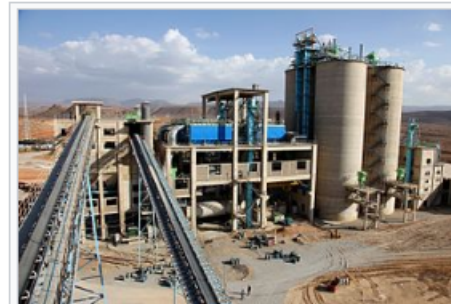
The National Cement Share Company of Ethiopia 's new plant in Dire Dawa ↗
