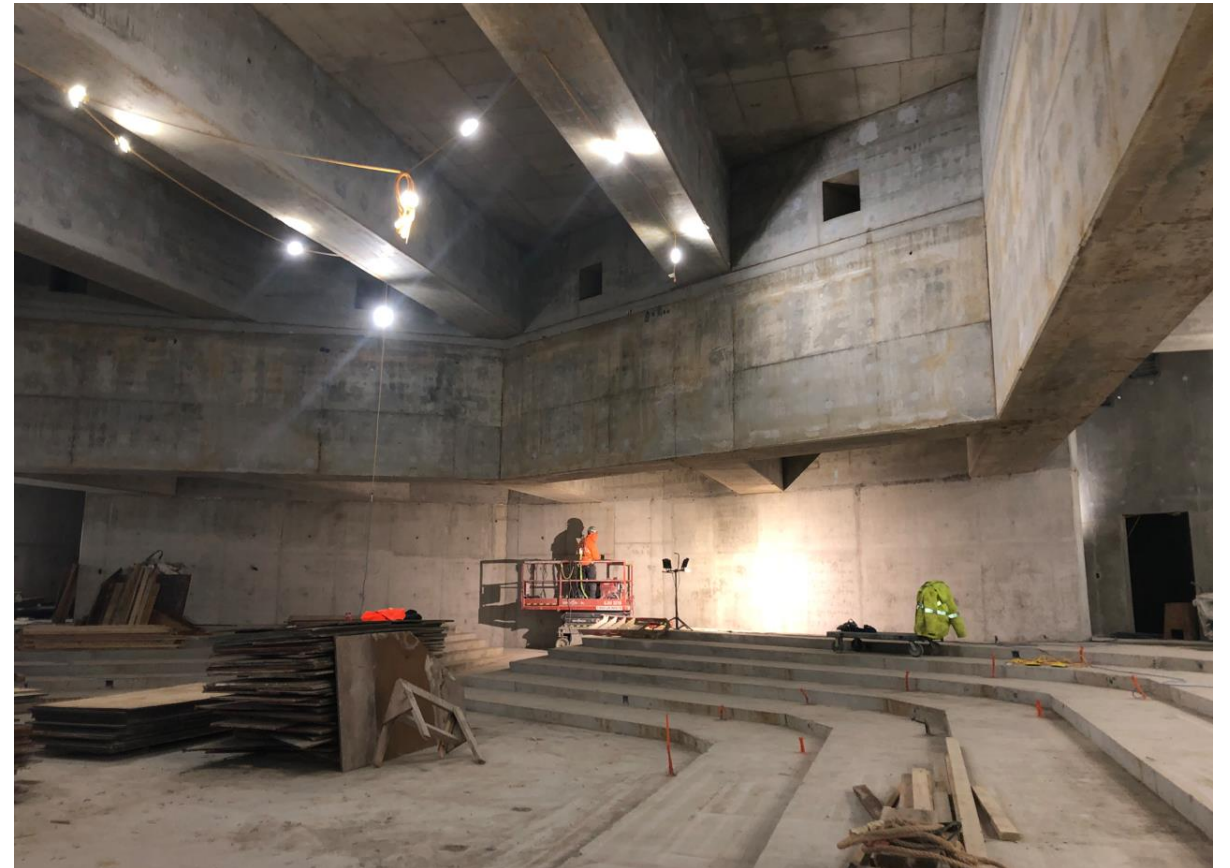
2 nd stage North South Roof Supporting beams
