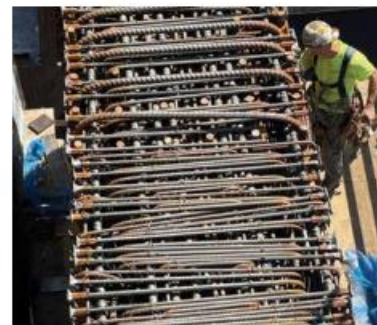
Fig. 8: Reinforcing bar density for this member was close to 800 lb/yd 3 . After this was built, the engineer changed bar sizes, bundled bars, and rearranged splices so there was access for concrete placement
