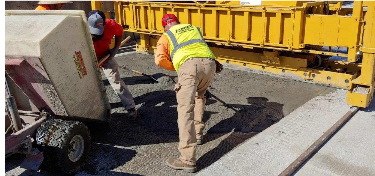
**Placing the UHPC Overlay with a Self-Propelled UHPC Paver.**
