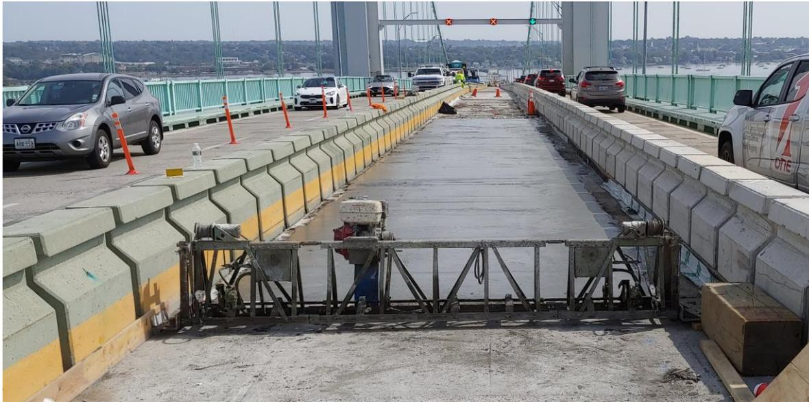
**Placing the UHPC Overlay with a Vibrating Bridge Deck Truss Screed.**
