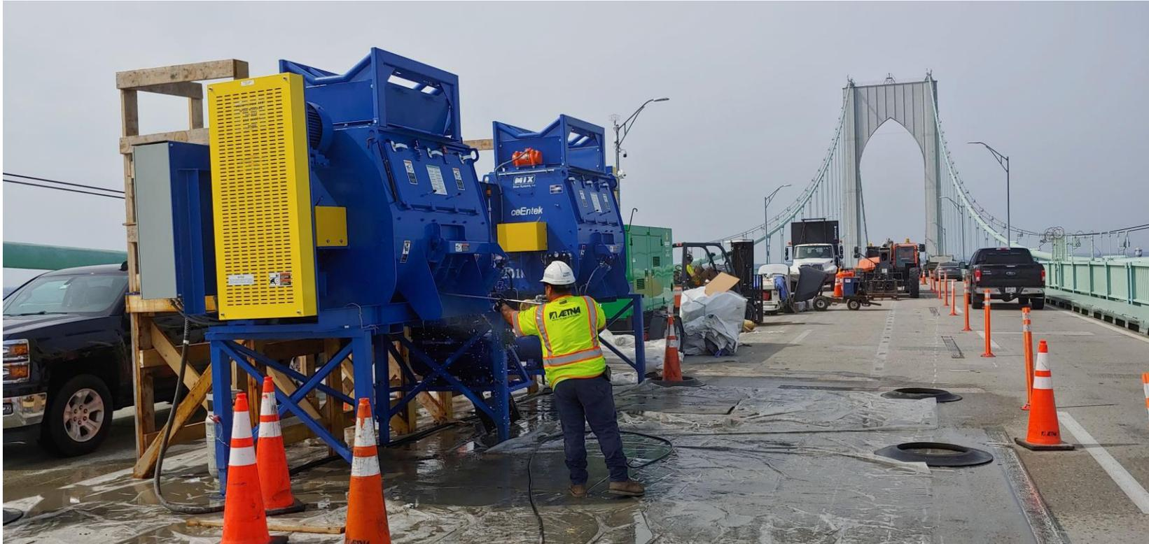
***Conducting a rehabilitation on a deck that is 200 ft in the air with slopes and cross-grades that are continuously moving (bending and twisting) from truck traffic, wind and equipment.***
