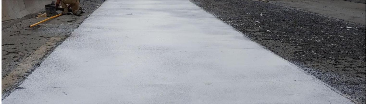
The finished surface of UHPC Overlay (L); Sprayed White Pigmented Curing Compound (Top); Covered with Wet burlap & Poly sheet (R).
