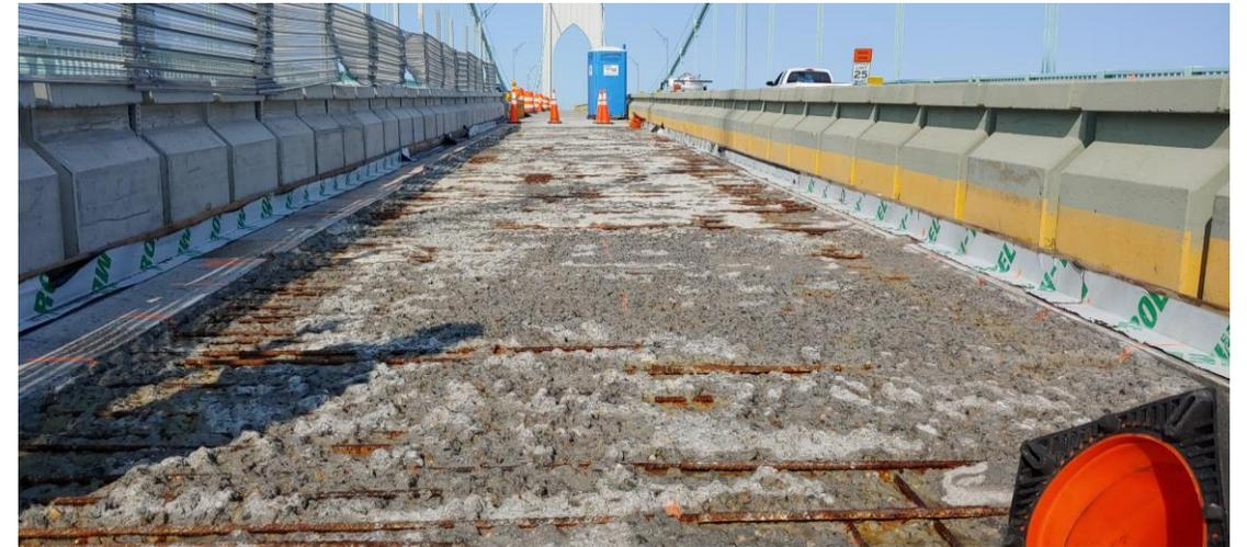
**Finished Surface after Hydro-Demolition of the Claiborne Pell Newport Suspension Bridge, RI**
