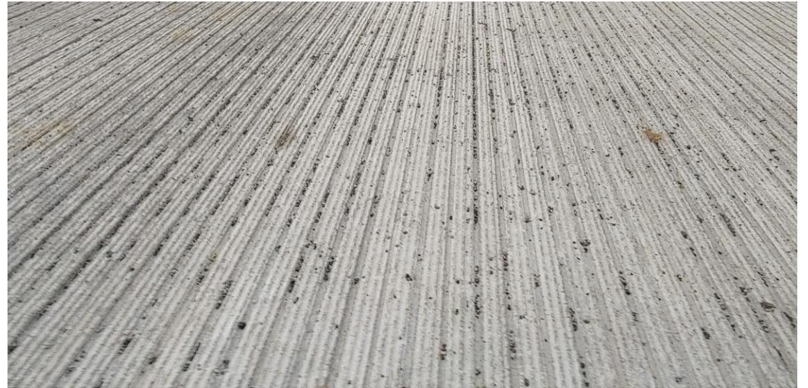
**UHPC Overlay Surface after Grinding & Grooving.**
