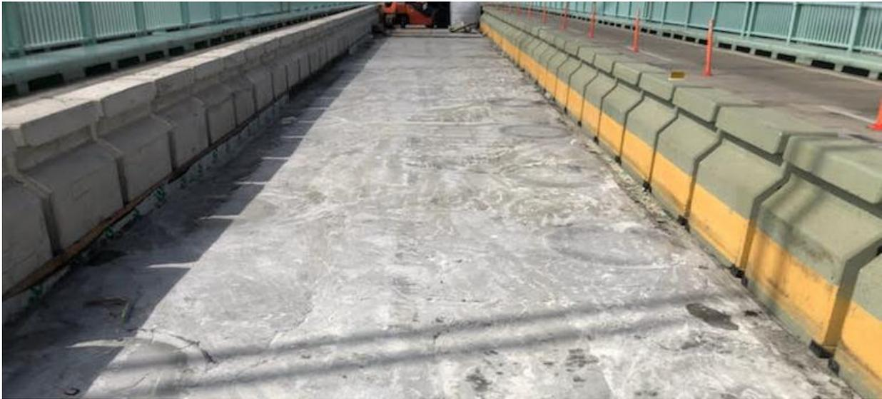
**Finished & Cured UHPC Overlay surface prior to Grinding & Grooving.**
