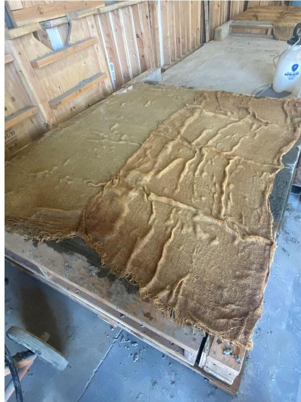
**Figure 6.** Covering the panel with wet burlap
