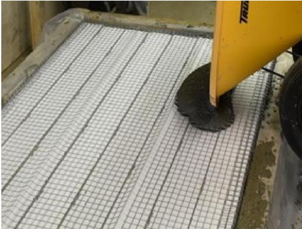
**Figure 3.** Pouring the top layer
