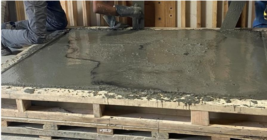
**Figure 5.** Finishing the top layer
