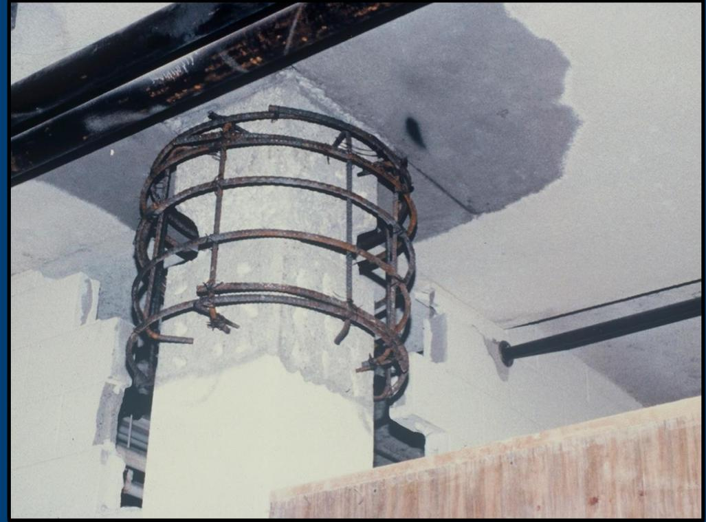
*Section enlargement of a column to increase slab punching shear capacity*
