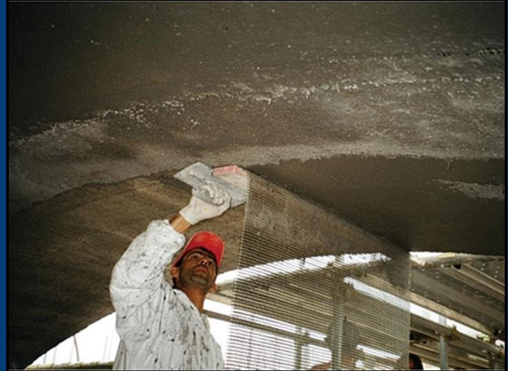
*Installation of FRCM on an arch*
