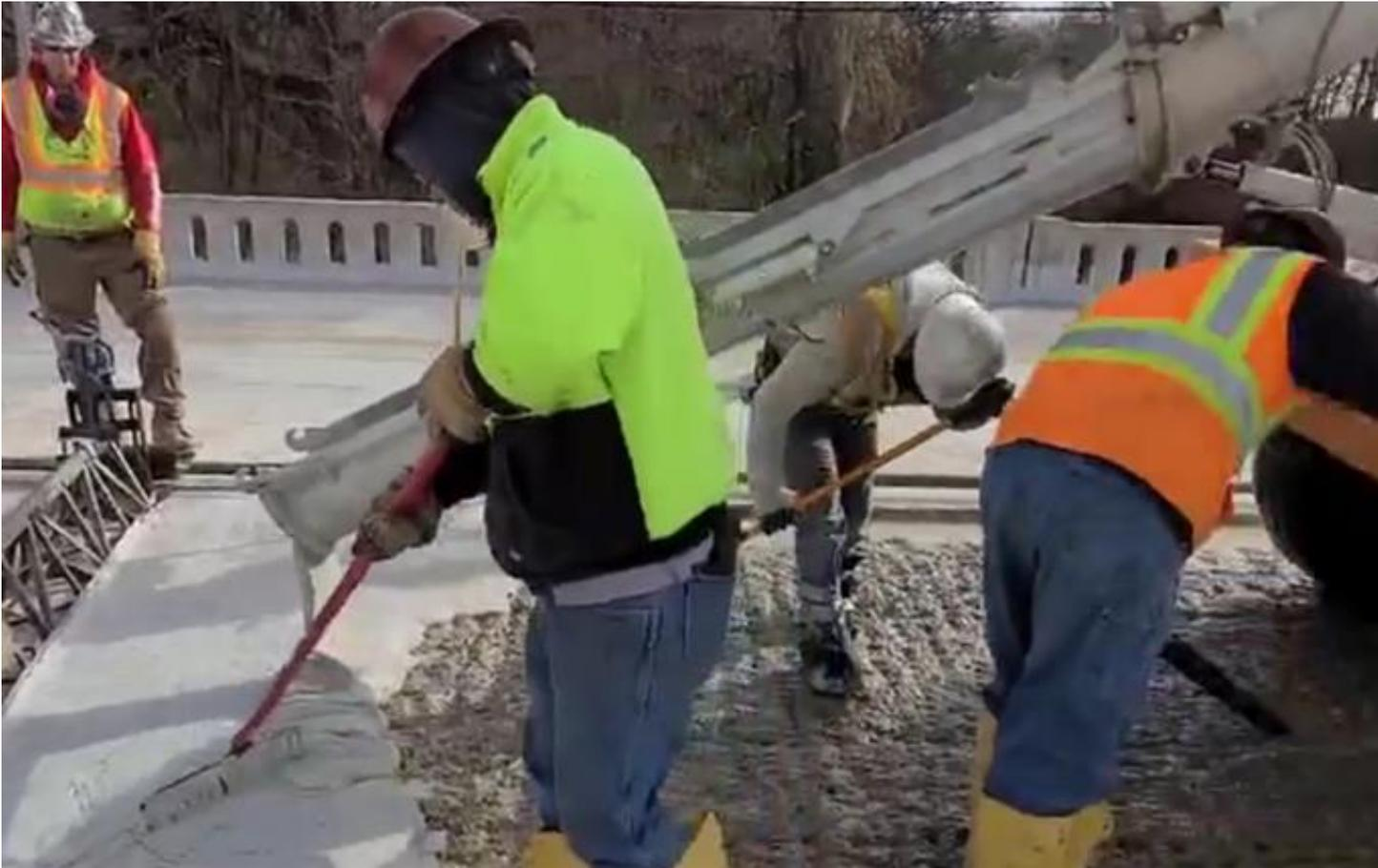
Directly discharging Steelike® UHPC onto bridge deck in front of screed.
