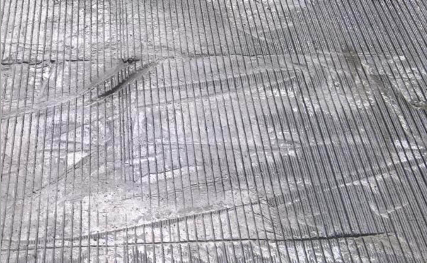
Impressions in final grinded and grooved surface from sheeting
