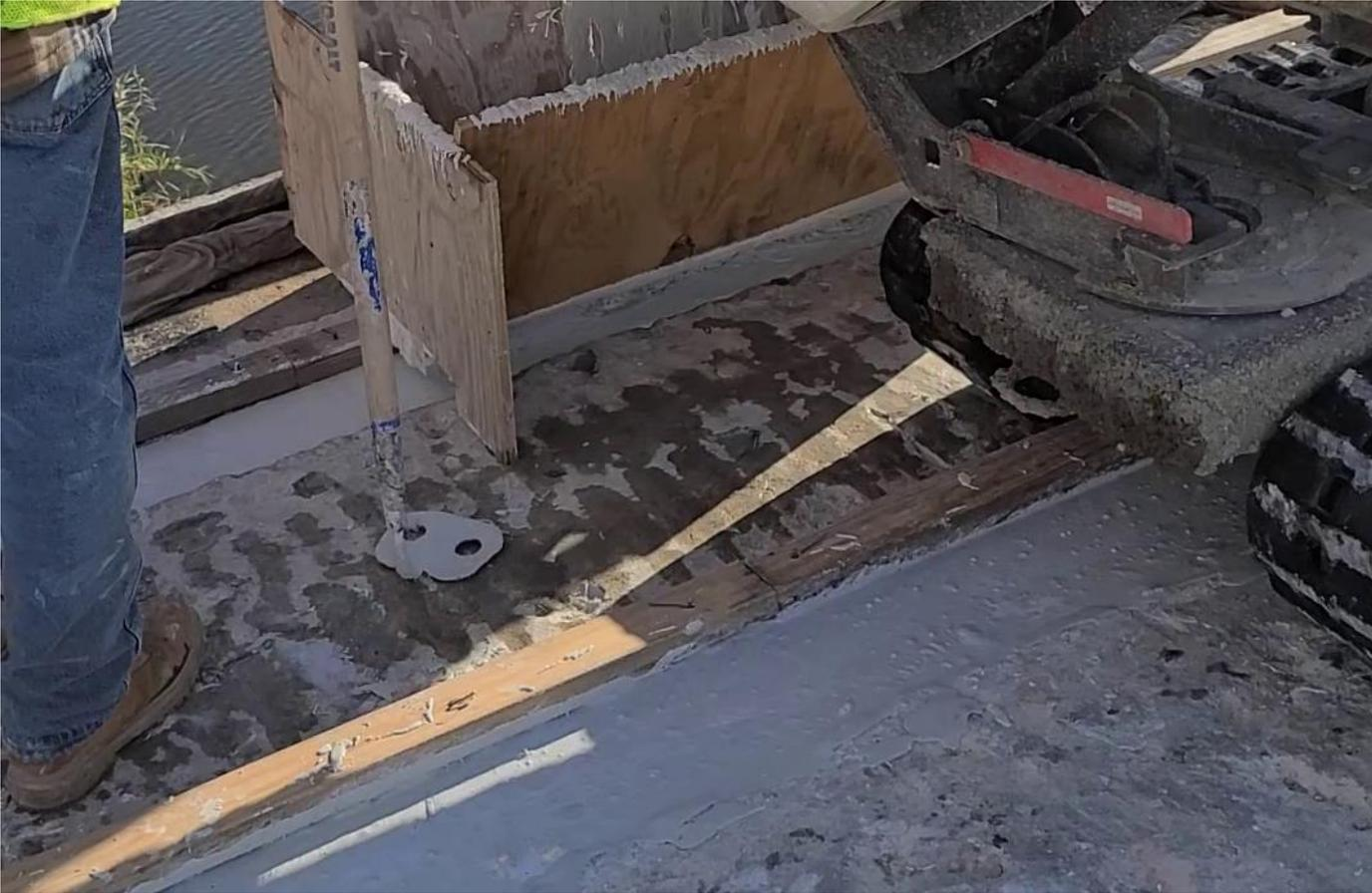
Placing Steelike® UHPC in longitudinal connections with no top forms
