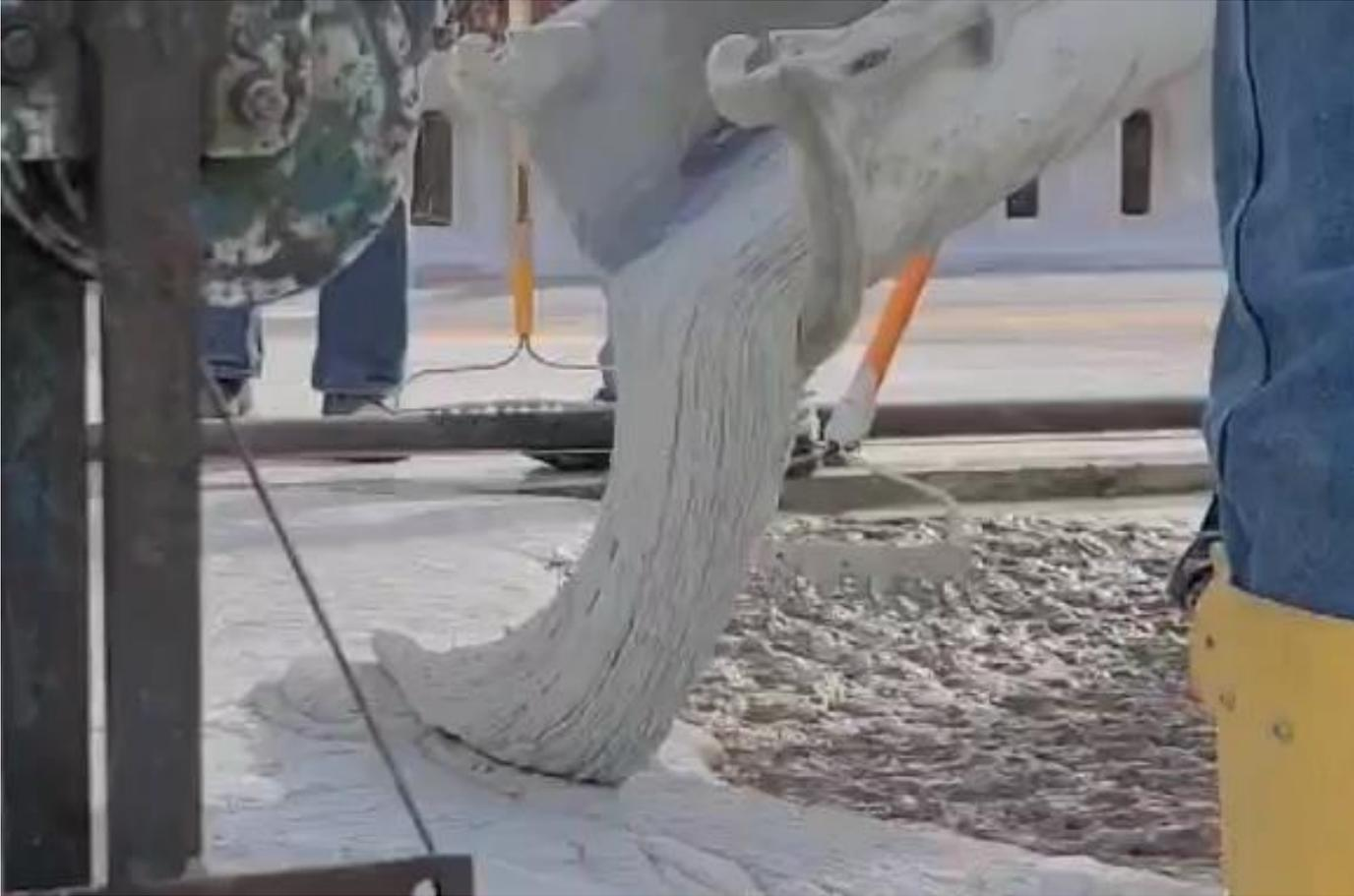
Directly discharging Steelike® UHPC onto bridge deck in front of screed.
