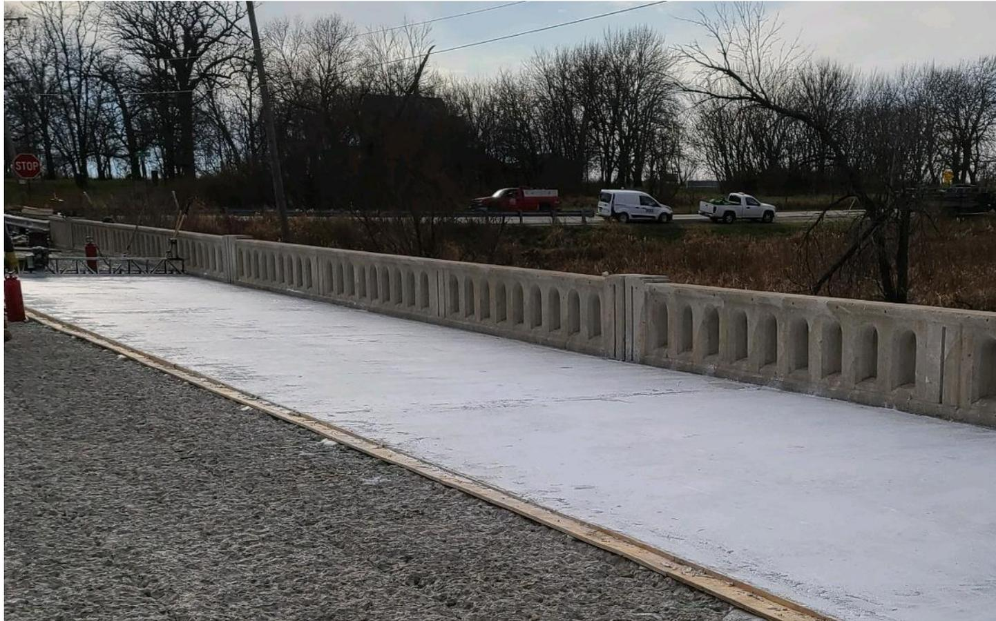
Curing Steelike® UHPC overlay without plastic sheeting.
