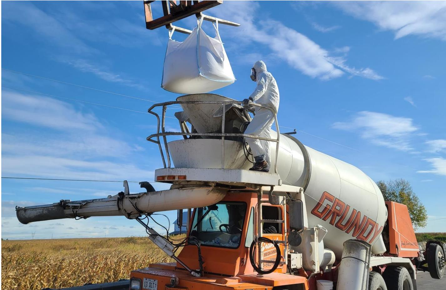
Mixing Steelike® UHPC in standard ready-mix truck
