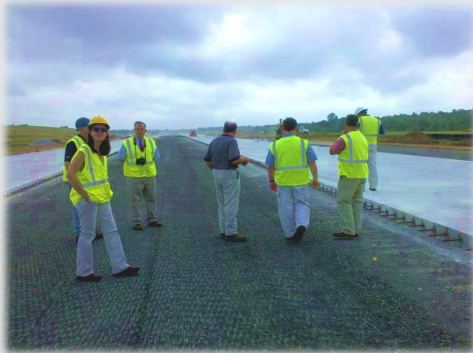
Lancaster County Airport Concrete Overlay of Asphalt
