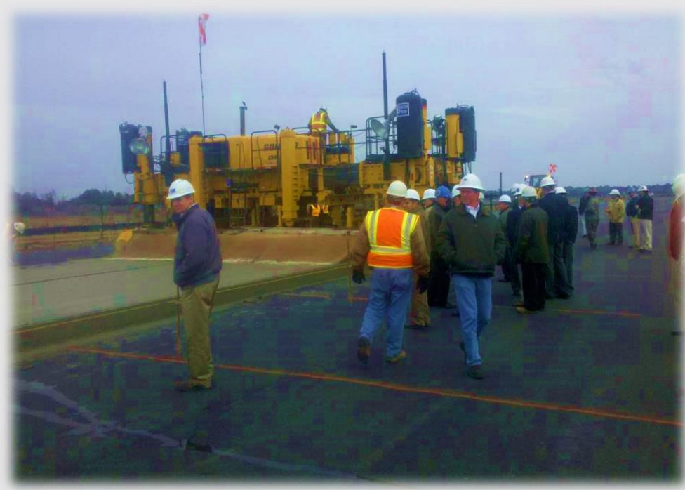
Charleston Exec Airport Concrete Overlay of Concrete
