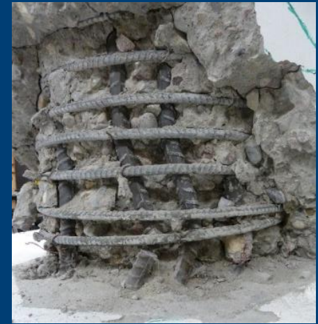
10.0% Drift Ratio (3 rd Rebar Rupture)
