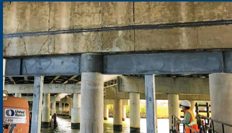
NSM TiABs Technology Used in San Jacinto River Bridge by TxDOT
