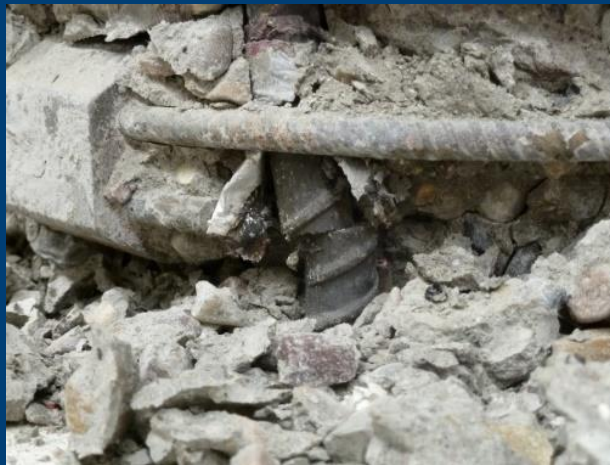
10.0% Drift Ratio (2 nd Rebar Rupture)
