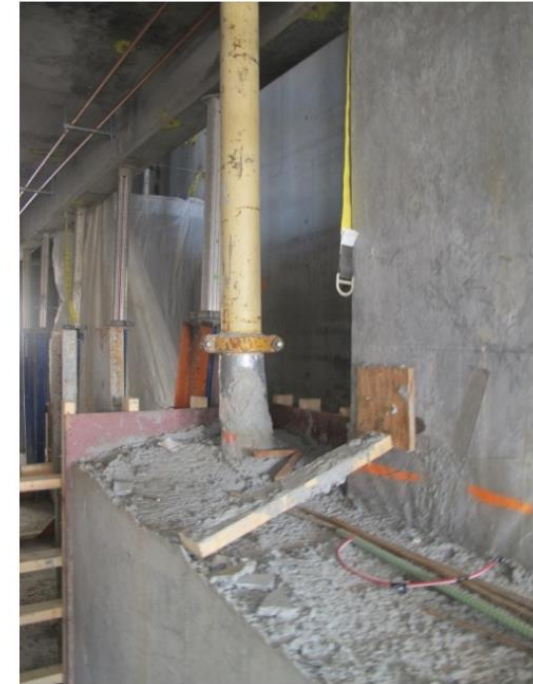
Vertical turn anchored in concrete
