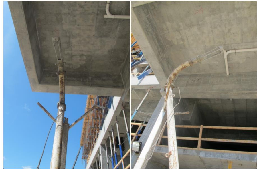
This discharge pipe sends the concrete back into the truck to be taken away. Notice the trap basket to catch the sponge ball
