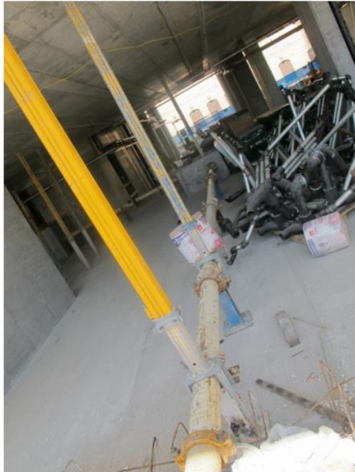
Horizontal Pipe line anchored to floor
