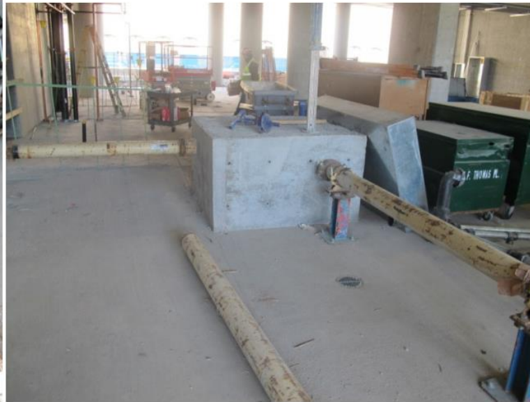
90° turn anchored in a concrete block
