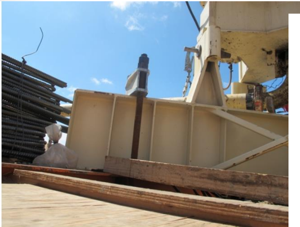
Base of Placing Boom attached to forming system at central core.
