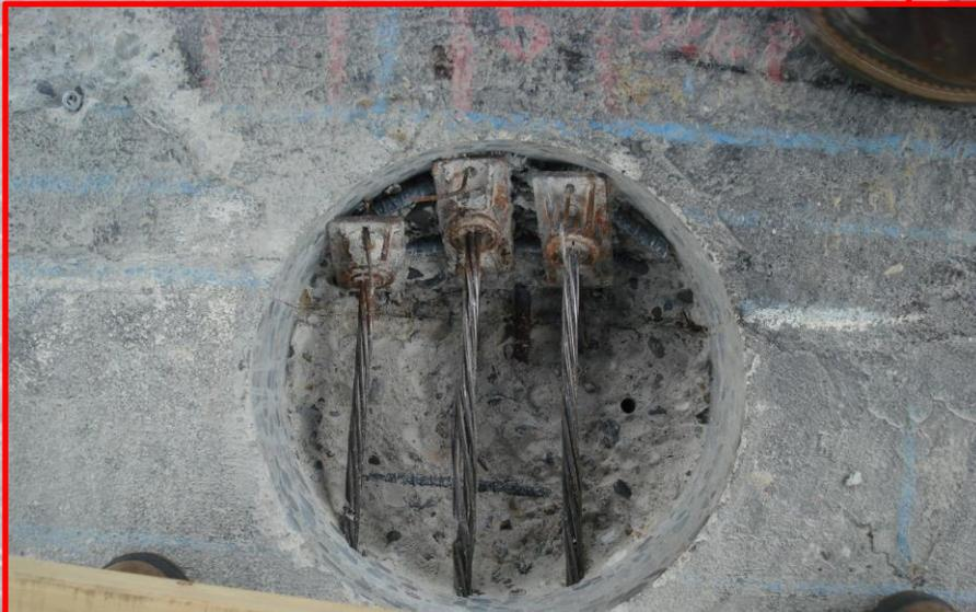
**Severed Anchors by Core Drilling**
