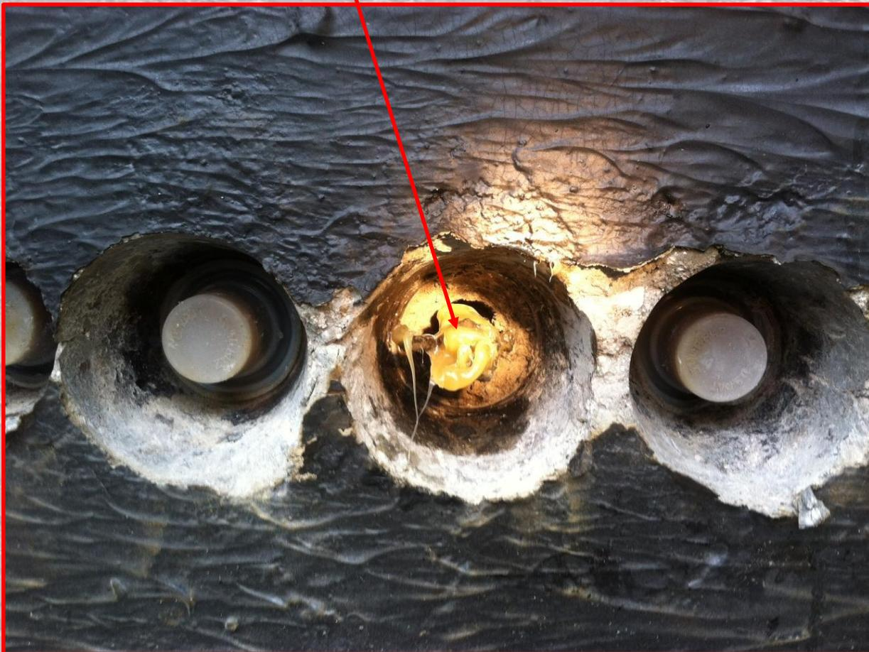
**Severe Corrosion of Wedges and Anchor**
