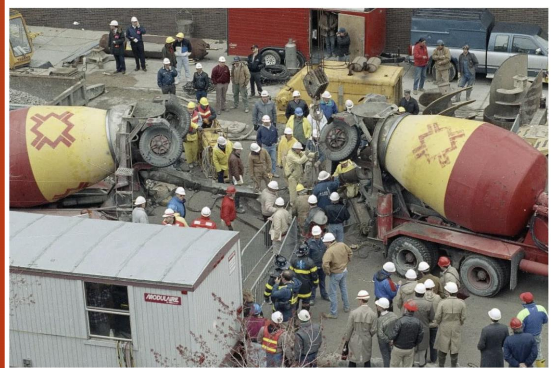
Workers prepare to pour cement into a shaft leading to a flooded tunnel to block the flow from the Chicago River on April 18, 1992, days after a leak caused the Loop Flood of 1992. | Charles Bennett / AP
