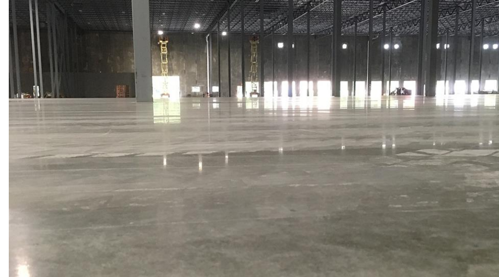
F.W. Webb Company, Londonderry, N.H. 40,000 joint-free slabs
