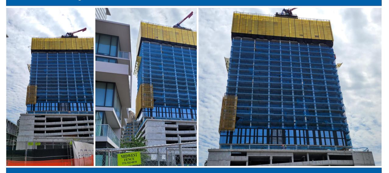
Worked with Lendlease to create a system to encapsulate the slab edge during window installation
