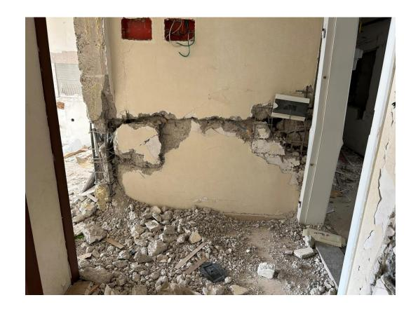
Lap splices at column and wall bases
