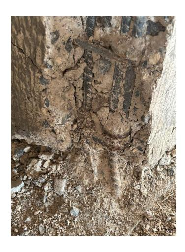
Offset-bent longitudinal bars (socalled "dog-Leg" detail) at the base of columns/walls
