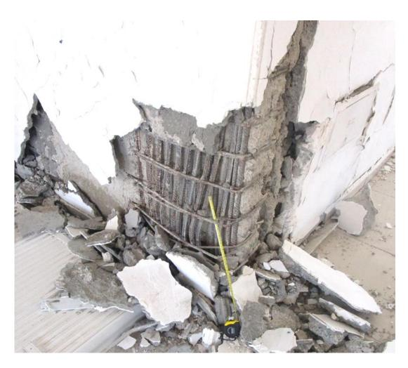
Concrete cover or longitudinal bar spacing smaller than required
