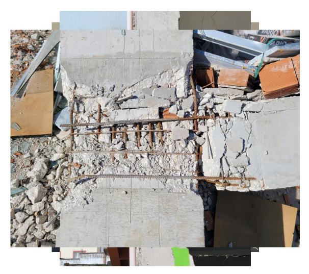
Unconfined beam bars in beamcolumn joints
