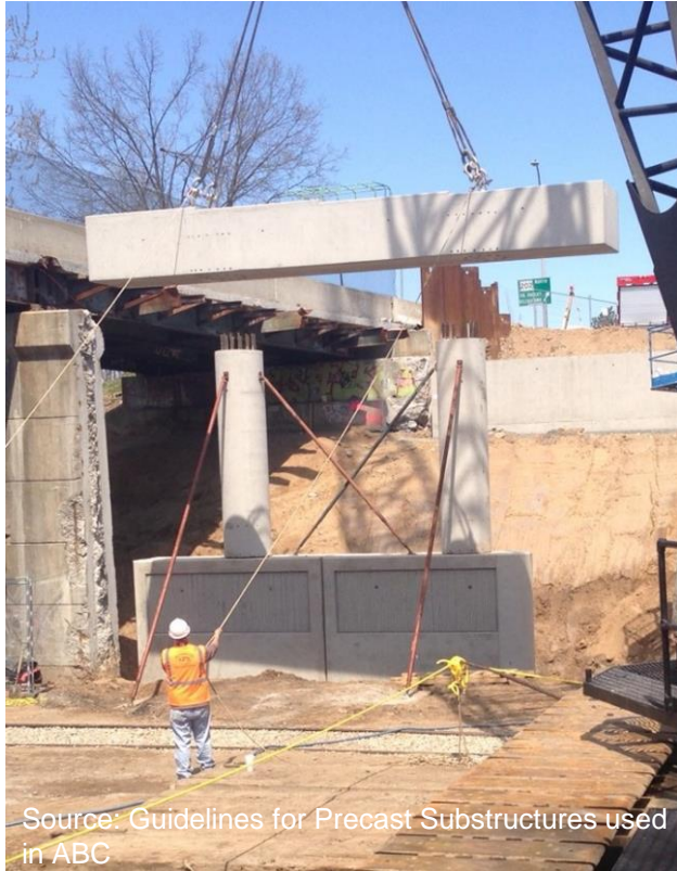
Route 202NB over B&M Railroad Holyoke, MA
