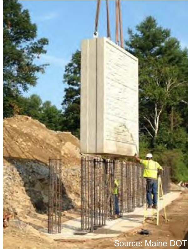
Route 1 Bridge over Route 236 Kittery, Maine
