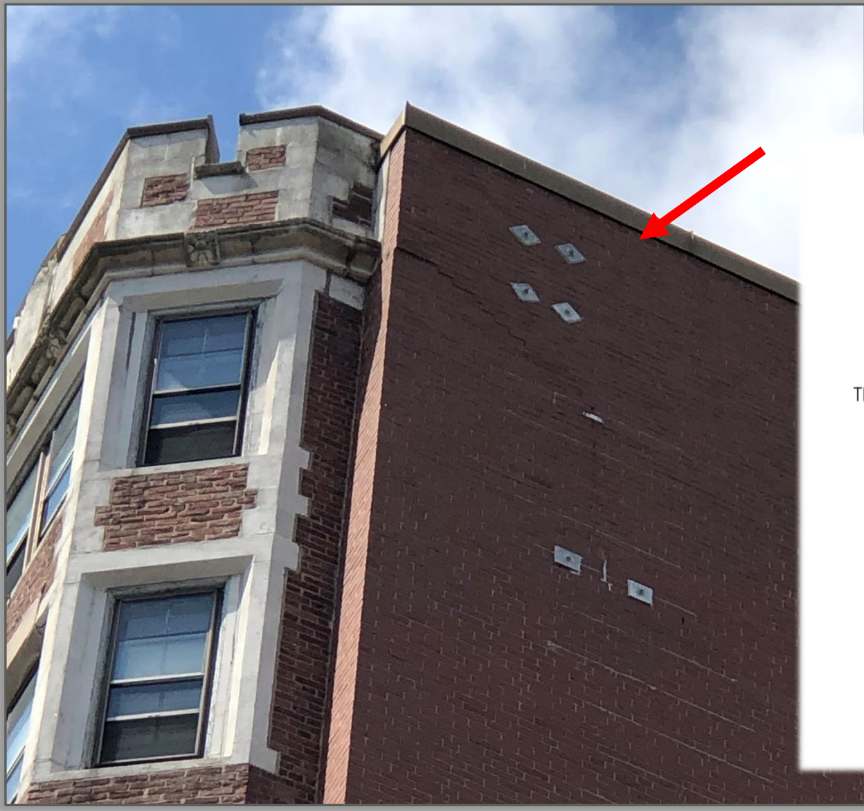
8 ANCHOR PLATE CONNECTION AT 10TH FLOOR
