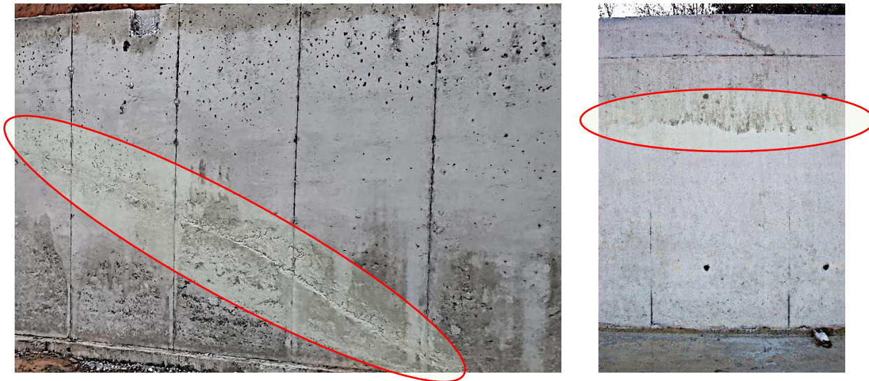
Strut Crossing Cold Joint in Stage Construction (Bayrak, 2020)
