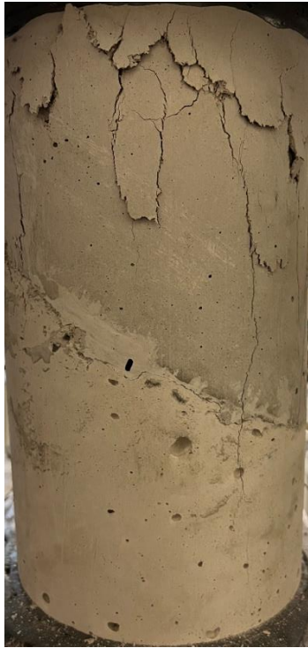
Crushing of concrete
