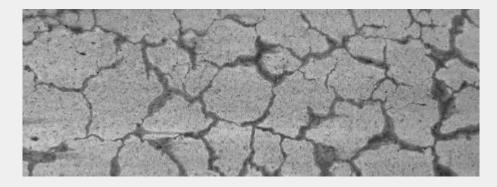
Chemical attack leads to the steady breakdown of concrete as it absorbs moisture.
