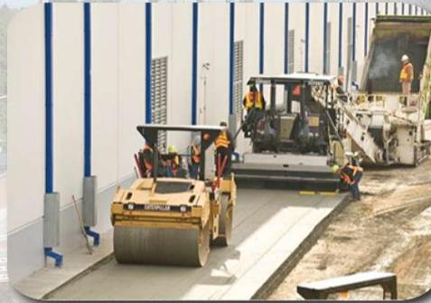
Roller-Compacted Concrete (RCC)
