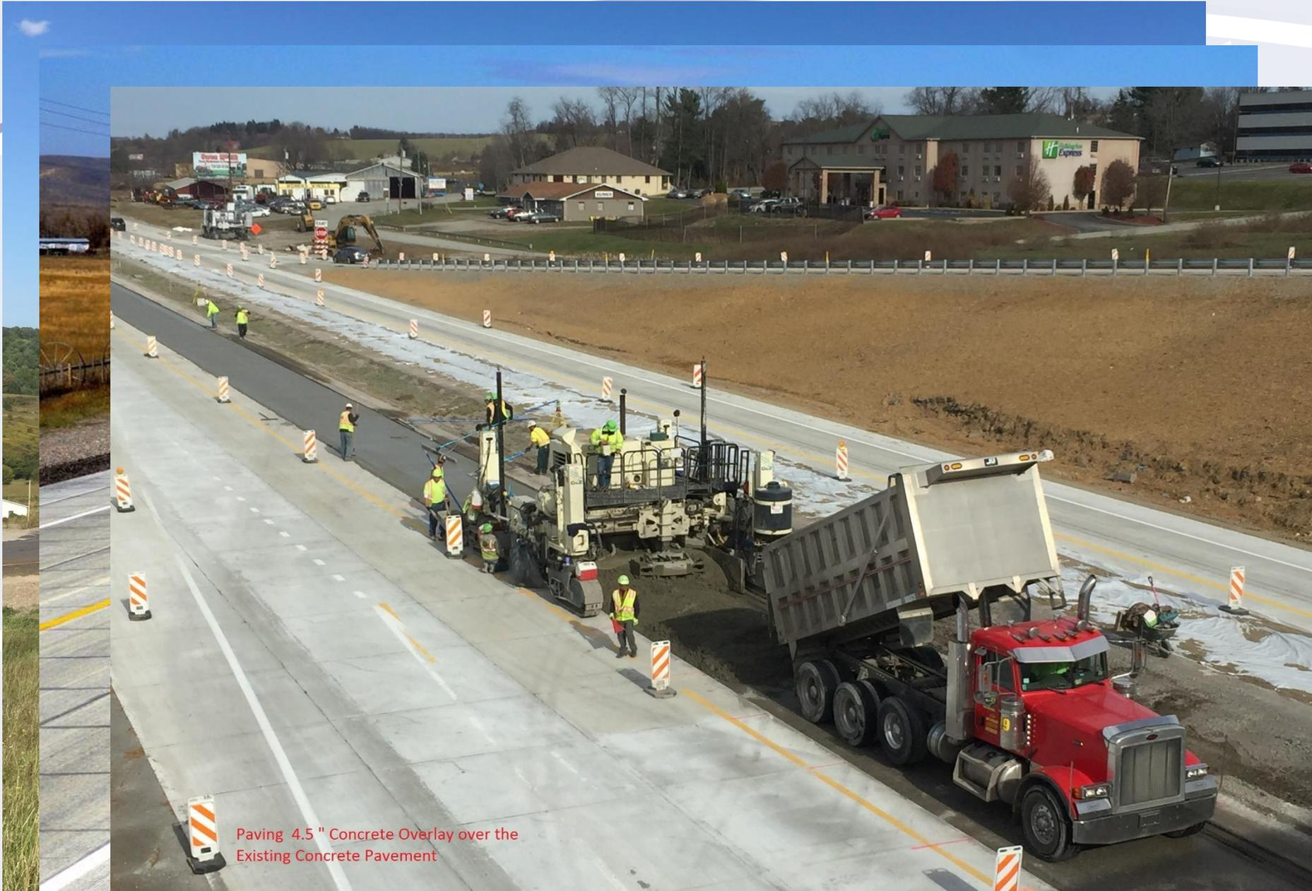
Paving 4.5" Concrete Overlay over the Existing Concrete Pavement
