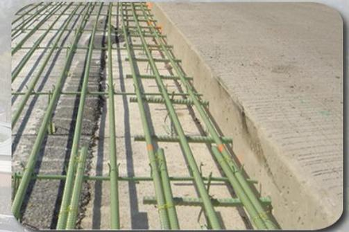
Continuously Reinforced Concrete Pavement (CRCP)
