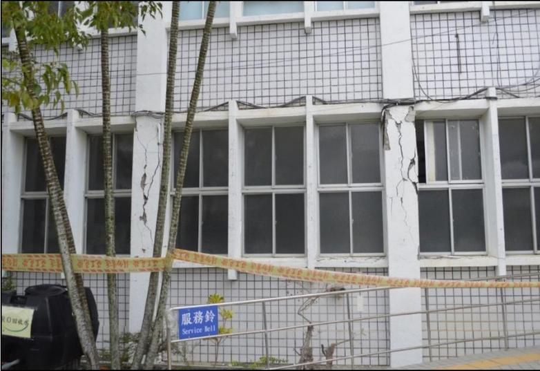
Vertical & Diagonal Cracking at
