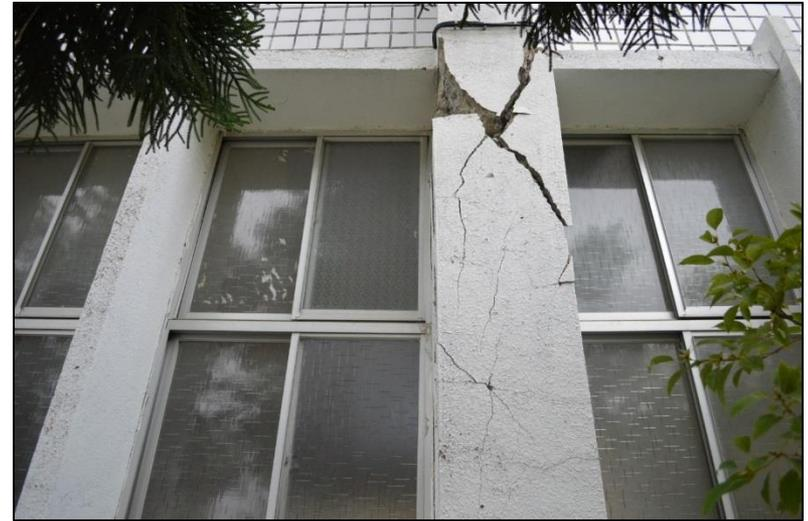
Diagonal Cracking at Column A9
