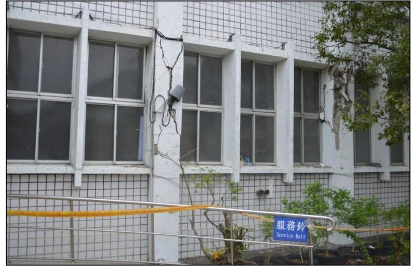
Vertical & Diagonal Cracking at Columns A7 & A8
