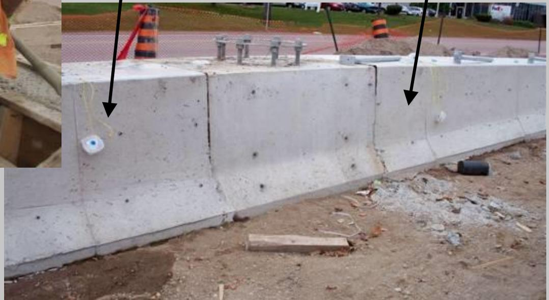
23 m<sup>3</sup> of each mix placed, 30 MPa, 60-100 mm (2.5-4 in.) slump
