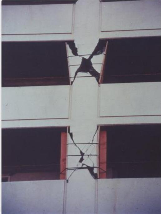
1994 Northridge earthquake, Champagne Tower, 16-story residential building, Santa Monica, CA, Typical X-shaped cracking in "short columns", photo credit: Comartin et al.
