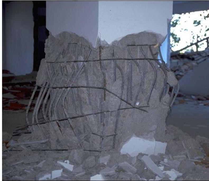
Two instances of column damage at the lap-splice location, 1999 Izmit, Turkey earthquake, photo credit: NISEE
