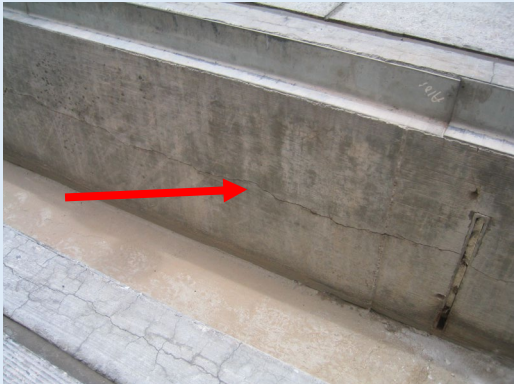
Expansion in base cracking fuel trench wall (2004)
