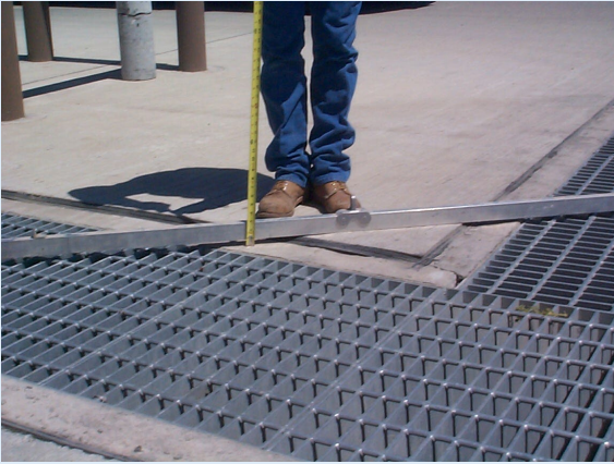
Heaving of apron on recycled base Fuel trench founded below recycled base.
