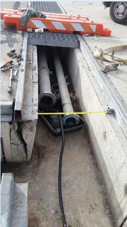
Heaving of apron on recycled base Fuel trench founded below recycled base.
