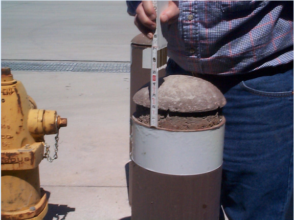
Concrete-filled bollard founded in recycled base
