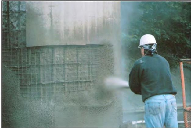
*“Concrete placed by a high velocity pneumatic projection from a nozzle.”*
