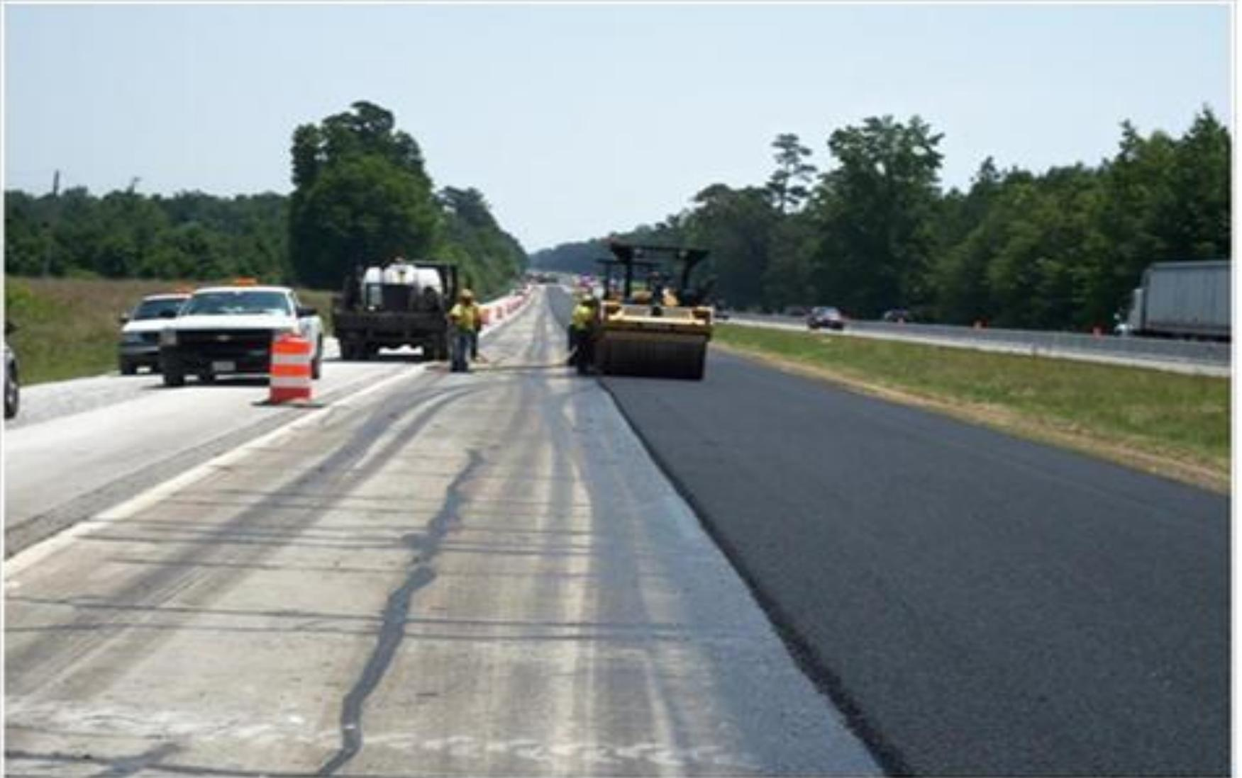
1 inch Asphalt Porous Friction Course (PFC)
