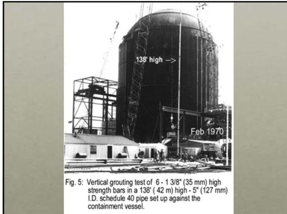
Fig. 5: Vertical grouting test of 6 - 1 3/8" (35 mm) high strength bars in a 138' (42 m) high - 5' (127 mm) I.D. schedule 40 pipe set up against the containment vessel.
