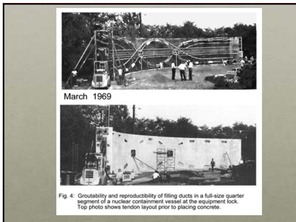
Fig. 4: Groutability and reproducibility of filling ducts in a full-size quarter segment of a nuclear containment vessel at the equipment lock. Top photo shows tendon layout prior to placing concrete.
