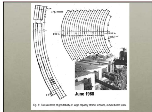
Fig. 3: Full-size tests of groutability of large capacity strand tendons, curved beam tests.
