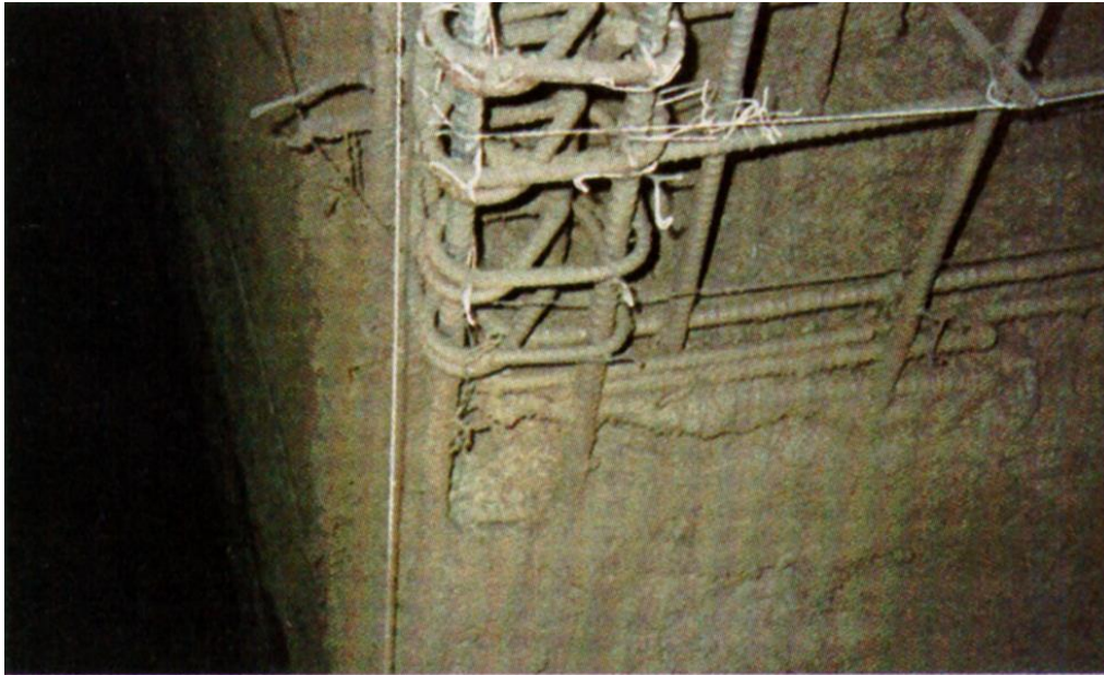
Figure 2: Ground wire delineates finish of a corner without restriction of nozzle trajectory.
