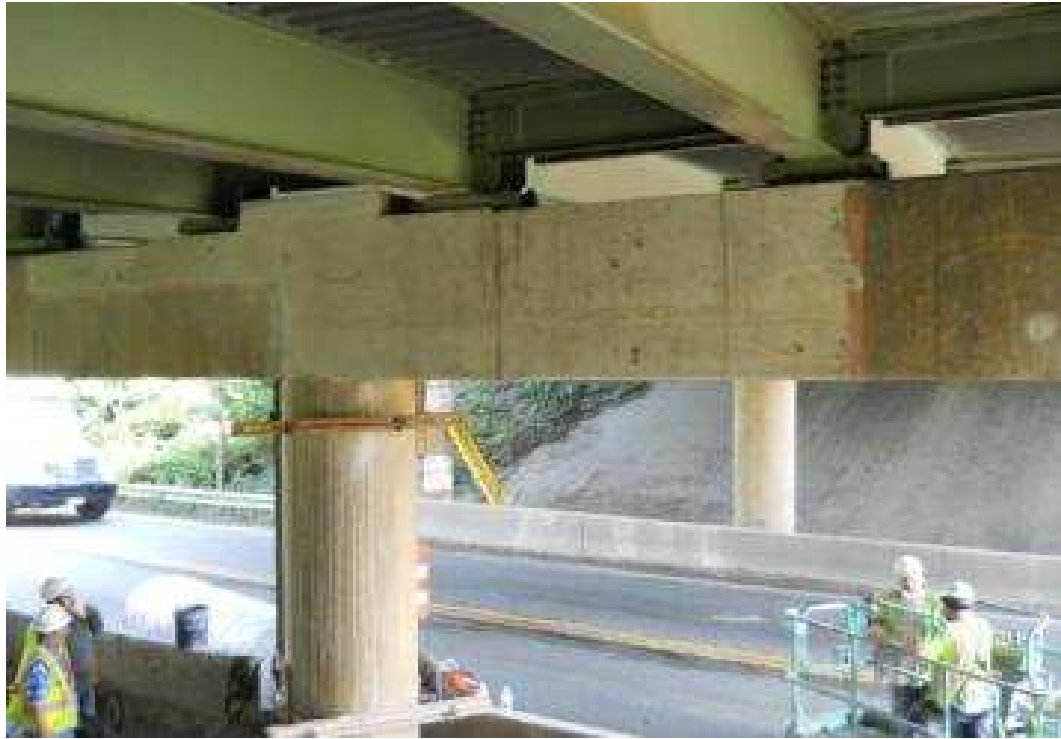
Completed pier cap
