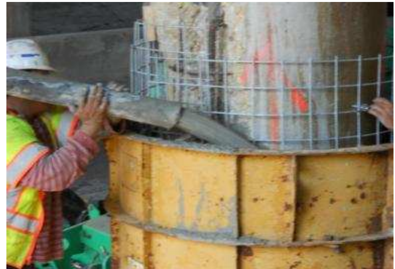
Increase in size of an existing column
