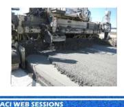
An optimized 2 lift with lower cementitious, SCMs, recycled concrete aggregate, etc. can easily reduce the  $CO_2$  by 50%.
