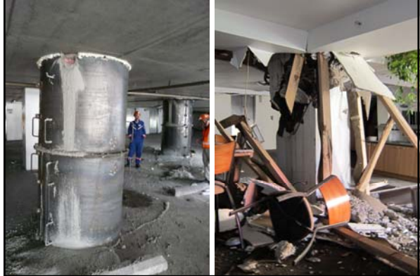
Stabilization - Level 10 Columns: March 5+
