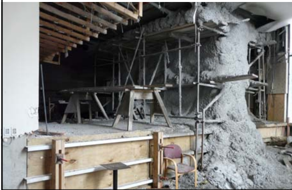
Shotcrete lobby wall: March 2-5
