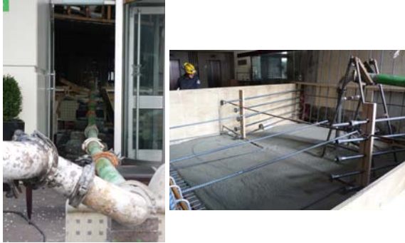
Pump concrete – east support: Feb 28
