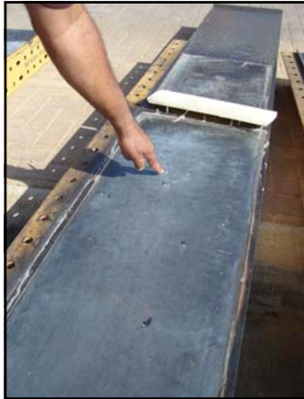
The side forms for the same mockup were also inspected. Note that James Hill is pointing to additional distinctively shaped dots of grout splash.
