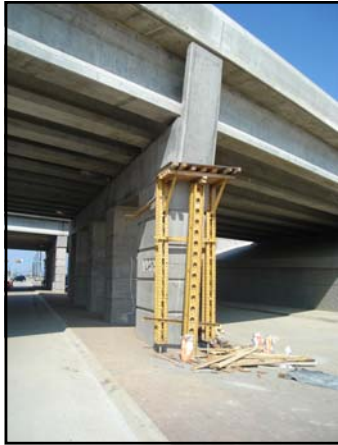
Adjacent to the mockup pour at the Coit Road Bridge is the recently stripped mask wall pour. Bug holes were noted on the surface.
