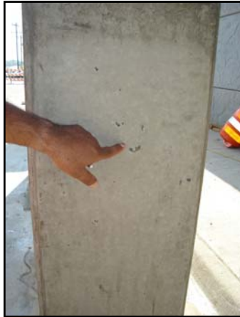
Showing a close-up view of the side of the same mockup surface and a mirror image of the distinctively shaped dots of hardened grout splash
