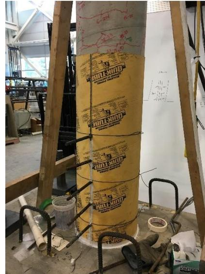
Formwork for pouring repair concrete
