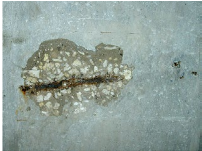
Fig. 1—Spalled concrete.
