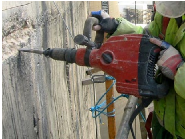
Fig. 2—Concrete removal.
