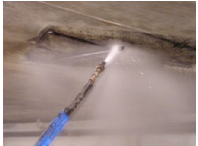
Fig. 4—Final surface cleaning after abrasive blasting.
