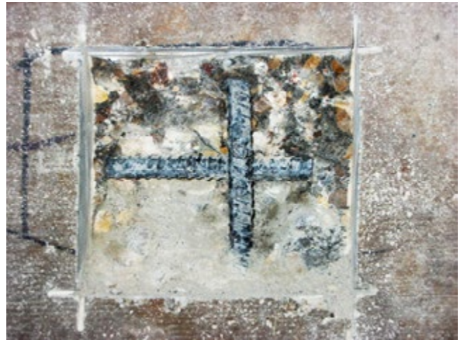
Fig. 5—Properly prepared surface.
