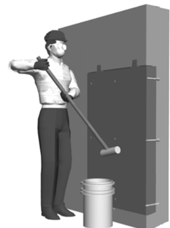
Fig. 4—Material placement: vertical application.
