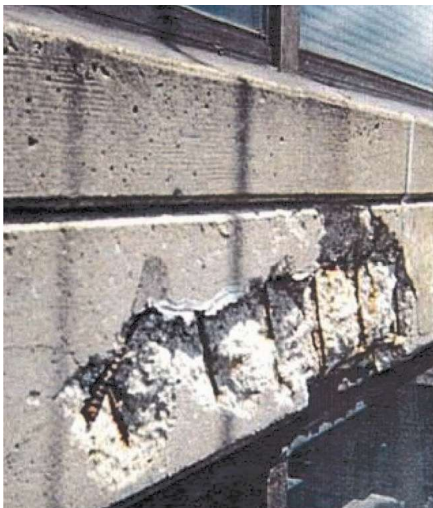
The accompanying guide to ACI 562 provides examples of actual concrete repair projects. In one example of a façade repair, the extent of concrete and steel deterioration was relatively minor. Spalling and delamination occurred mostly where reinforcing bars were placed too close to the surface and located in carbonated concrete. Photo courtesy of ACI.
