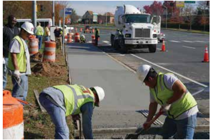
Concrete placement in Montgomery County, MD, trial of various SCM mixtures
