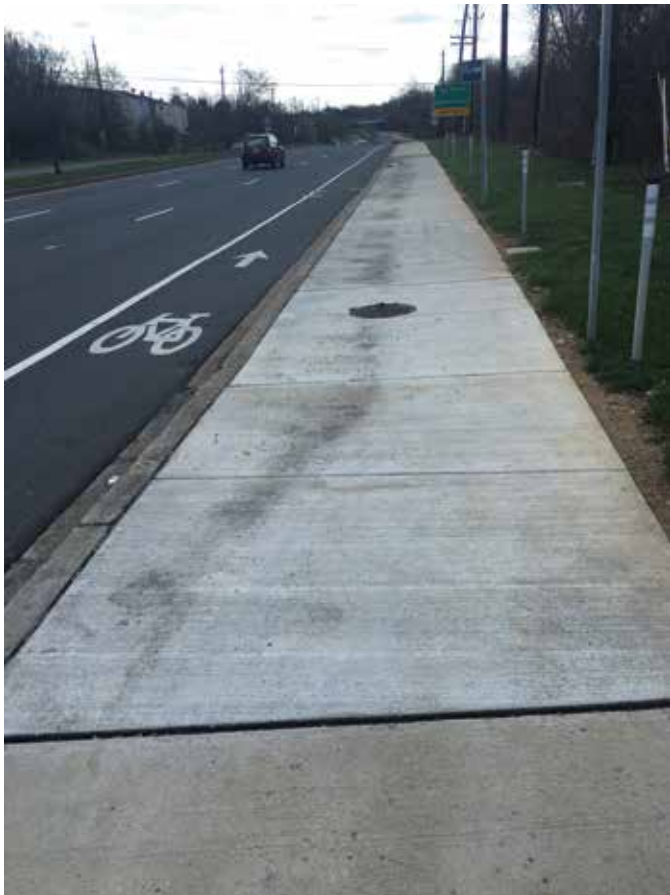
Slag cement sidewalks after a winter in service. Dark marks are temporary due to melting snow and ice
