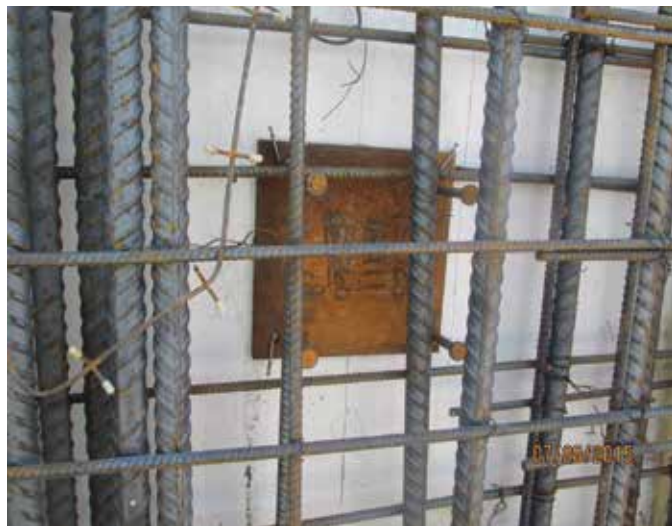
Fig. 6: Embed plates require small diameter holes for installation on wall form
