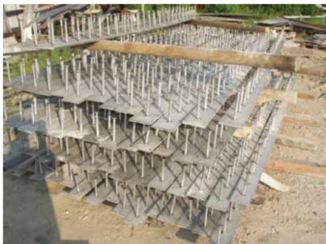
Fig. 8: Embeds must be stored in a designated area and supported on cribbing or pallets. In this example, several of the embed plates are curved, warped, or twisted. Slight imperfections can be corrected during installation once embeds are nailed in place. Note, however, that these plates lack nail holes. If adequate corrections cannot be made, deformed embeds should not be used
