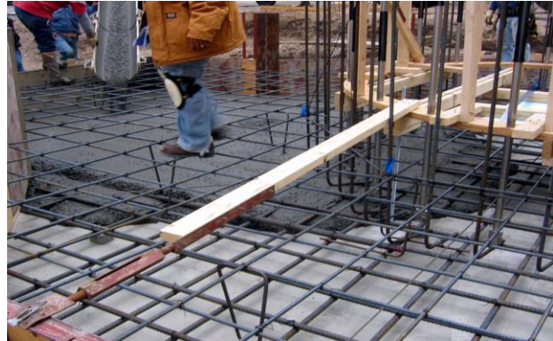
Fig. 7 Self-Consolidating High Percentage Silica Fume Concrete
