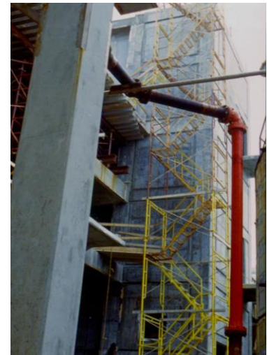
Fig. 3 Chemical Storage Building
