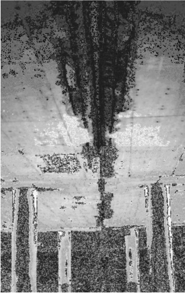
Fig. 2.9—Corrosion related damage under leaking longitudinal deck joint.
