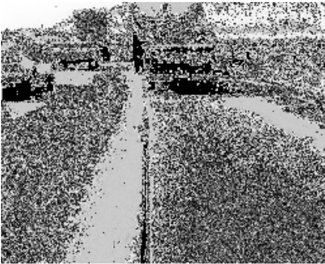
Fig. 2.7—Longitudinal view showing proximity of wheel path to joint.
