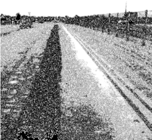
Fig. 2.7—Longitudinal view showing proximity of wheel path to joint.
