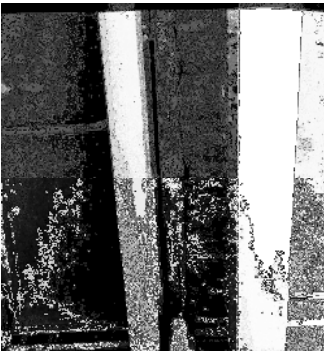
Fig. 2.9—Corrosion related damage under leaking longitudinal deck joint.
